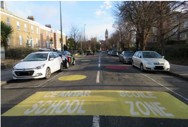
Image 5: Example road surface sign for School Zone, Leinster Road, Rathmines, Dublin 6
