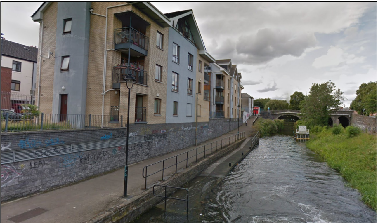
Figure 3: Existing Site Layout Showing Tow Path, Adjacent Residential Properties & Jetty
