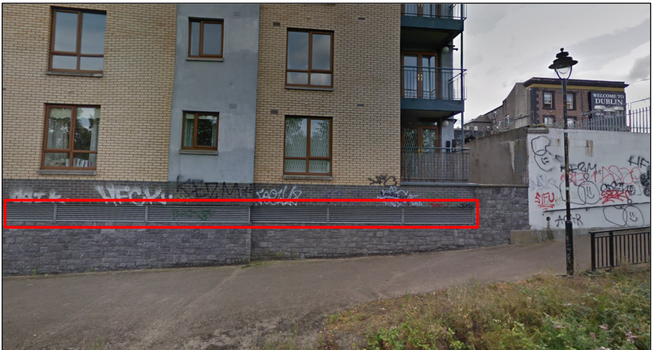
Figure 7: Existing Apartments Blocks Basement Vents Fronting Tow Path
