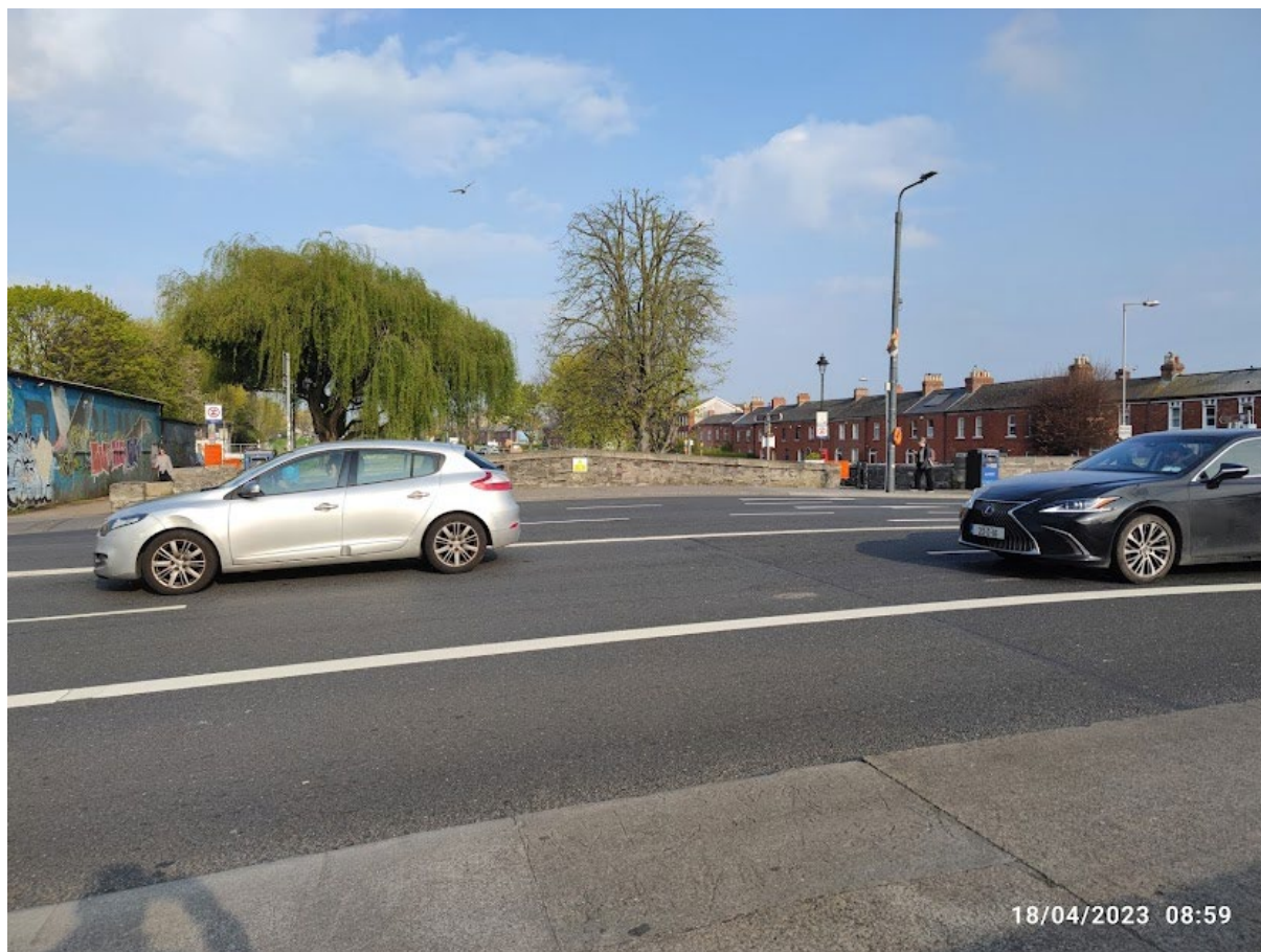
Figure 5.15. Binns Bridge (view from the sidewalk).
