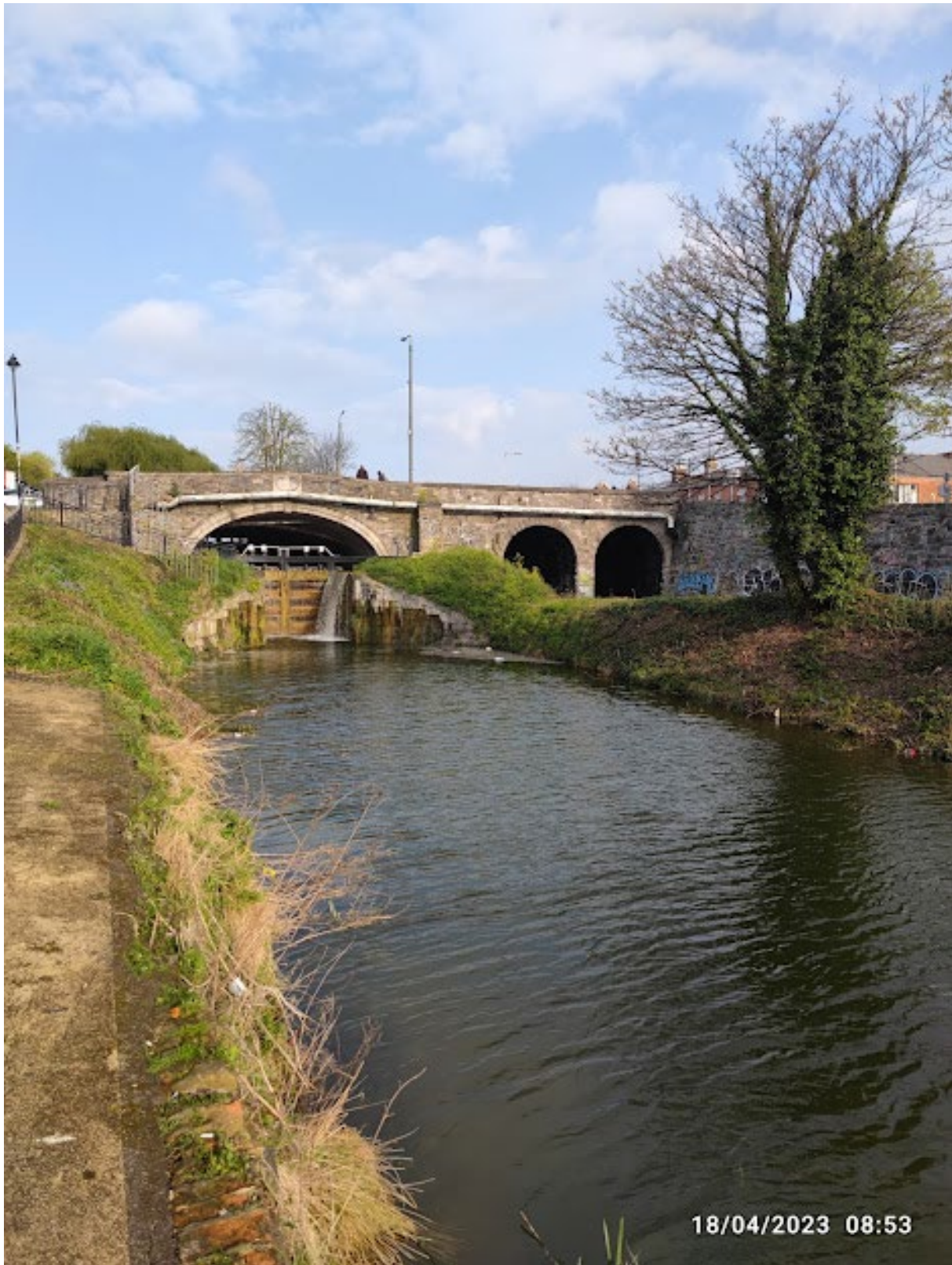
Figure 5.13. Grassy verges present near the bridge.
