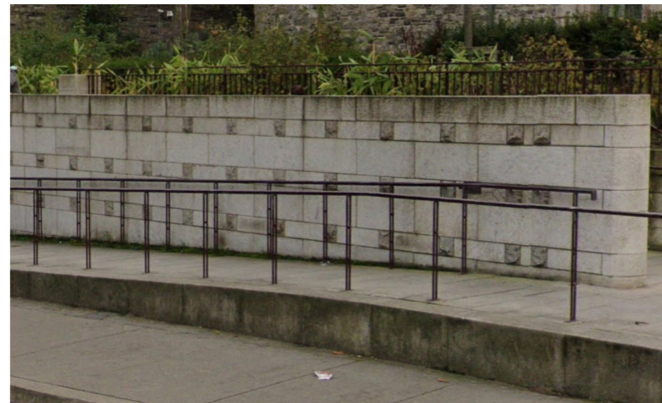
Fig 38. Contemporary expression (St Luke's, St Luke's Avenue) : Ashlar masonry detailing - stone should not be thin cladding at critical junctions i.e. steps should be solid not made up in sections
