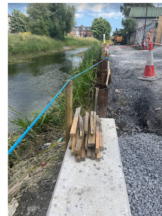
Fig 8. Capping beam to sheet piling
