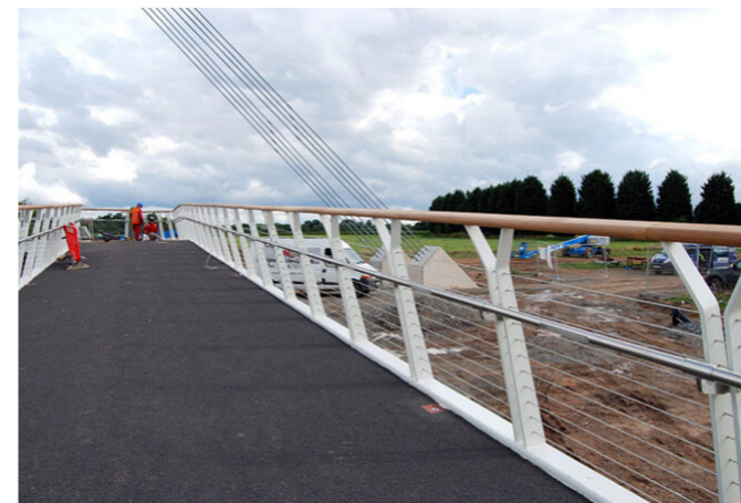
Fig 43. Cable type edge guarding: Example of railing references to maintain openness whilst meeting regulatory requirements. Existing railing at the Jetty structure are simple and open and provide precedent for new railings at the lock chamber edge.
