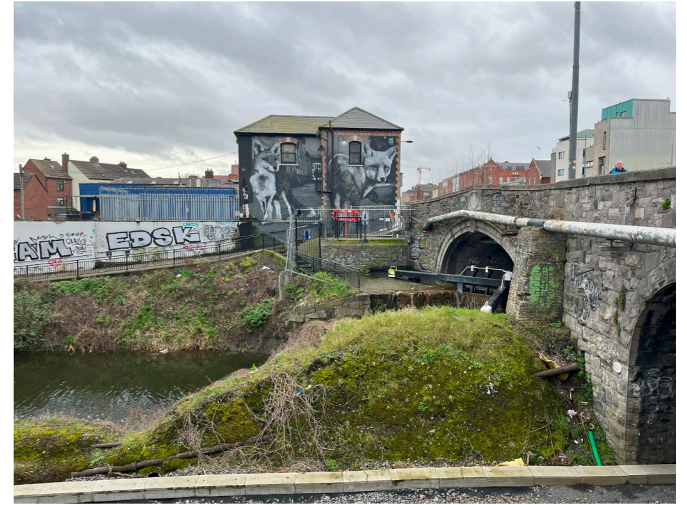
Fig 25. View southwards towards existing ramp transition.
