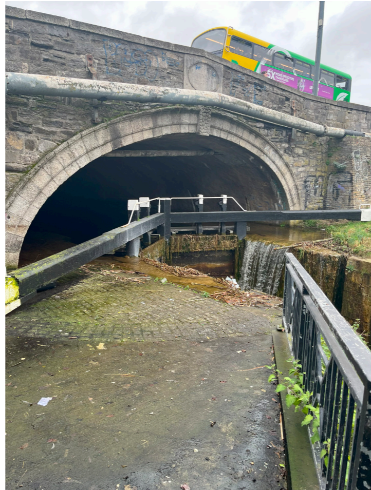
Fig 24. Lock chamber gate with balance beam.
