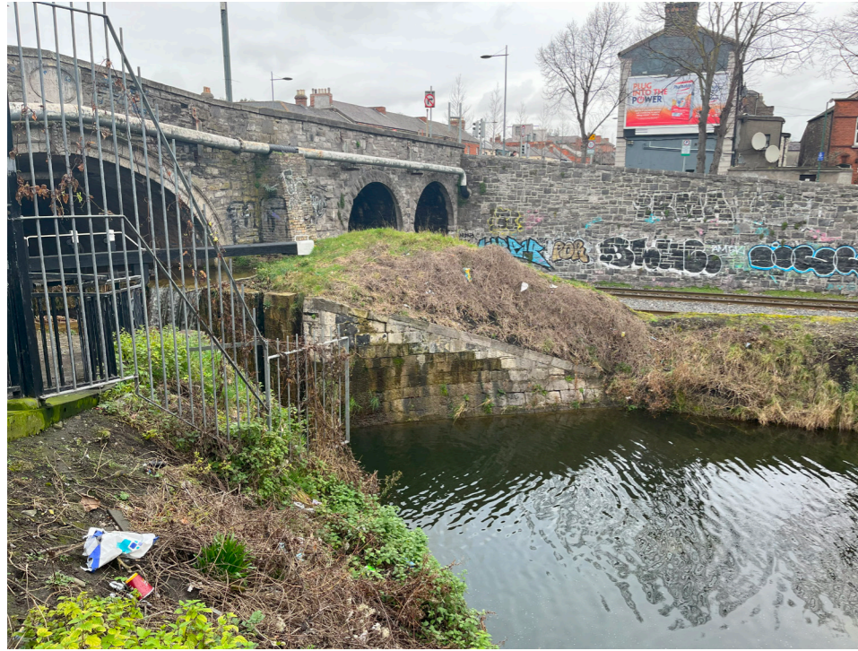
Fig 22. View to wing wall on northern canal embankment.
