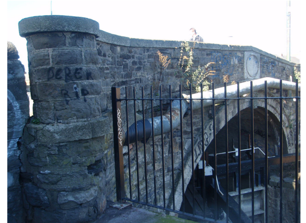
Fig 19. View towards bridge from top of ramp.
