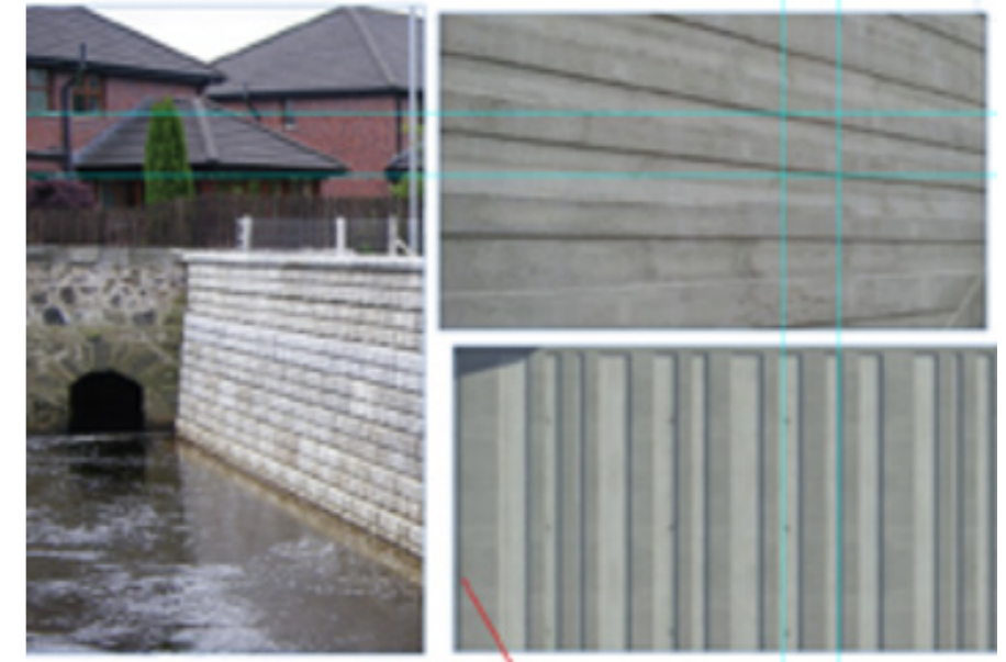
Fig 39. Alternative Option 1 – Concrete facing : Potentially incongruous to surroundings. There is a concern that longterm it will not weather well.
