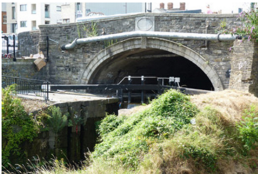
Fig 1. Binns Bridge (protected structure) view from northern embankment.
