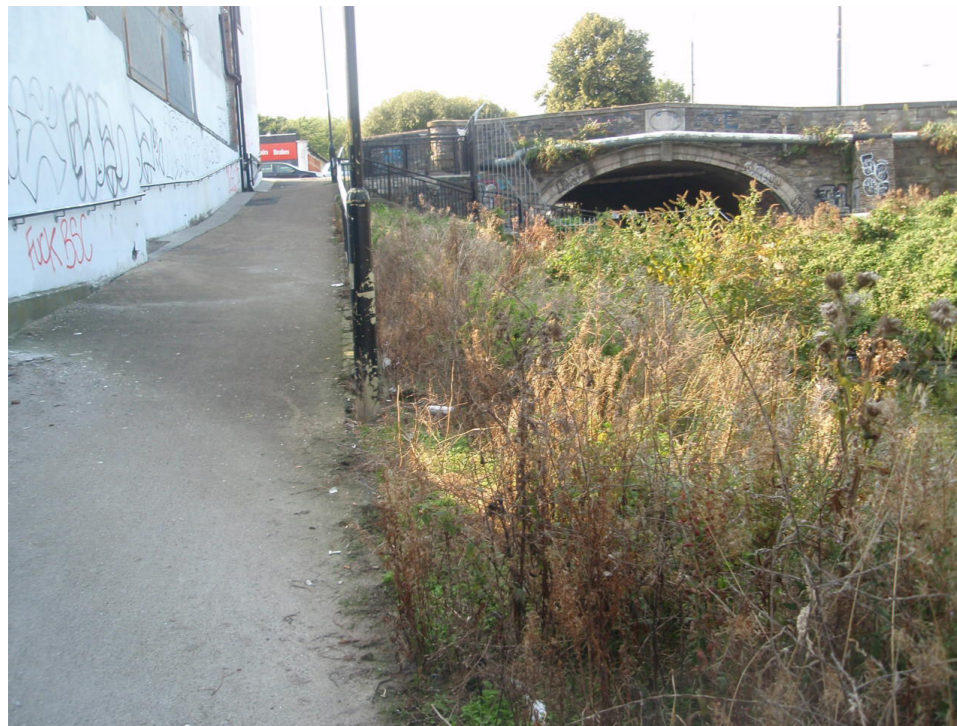
Fig 23. View along ramped tow-path.
