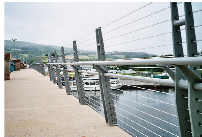
Fig 43. Cable type edge guarding: Example of railing references to maintain openness whilst meeting regulatory requirements. Existing railing at the Jetty structure are simple and open and provide precedent for new railings at the lock chamber edge.
