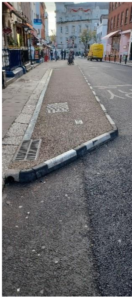
Image 11: Example path buildout on South William Street, Dublin 2
