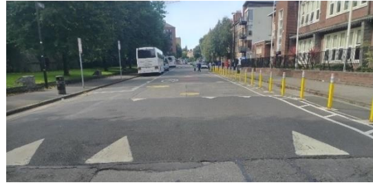
Image 9: Example speed ramp, Cook Street, Dublin 8
