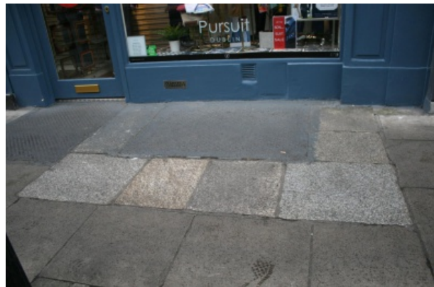
Feature Number: 14 - Original survey photo taken in 2019 of keg drop outside 14 Duke Street.
