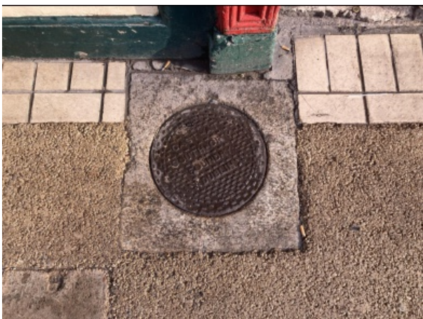
Feature Number: 48 - Granite slab with coal hole at 8-9 Anne Street South
