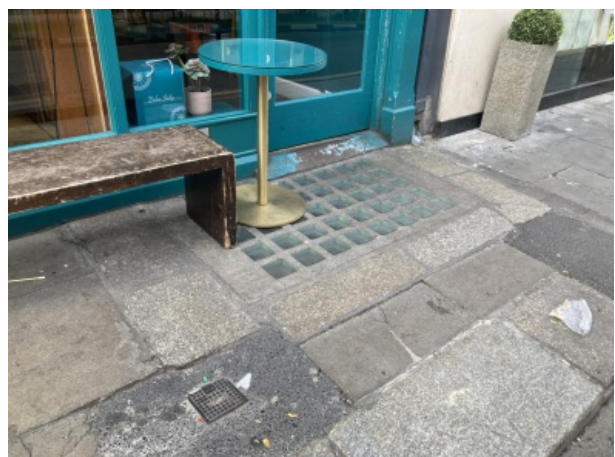
Feature Number: 36 - Lightwell, 20 Anne Street South
