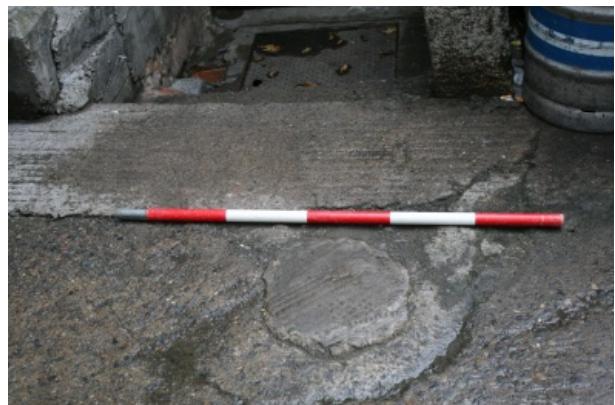
Feature Number: 66 - Possible coal hole cover at the Annes Lane access to 44 Grafton Street
