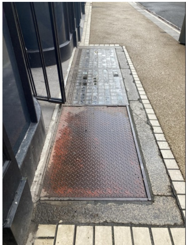
Feature Number: 53 - wo lightwells & metal door set in granite, 1 Anne Street South
