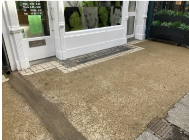
Feature Number: 52 - Lightwell, 4 Anne Street South
