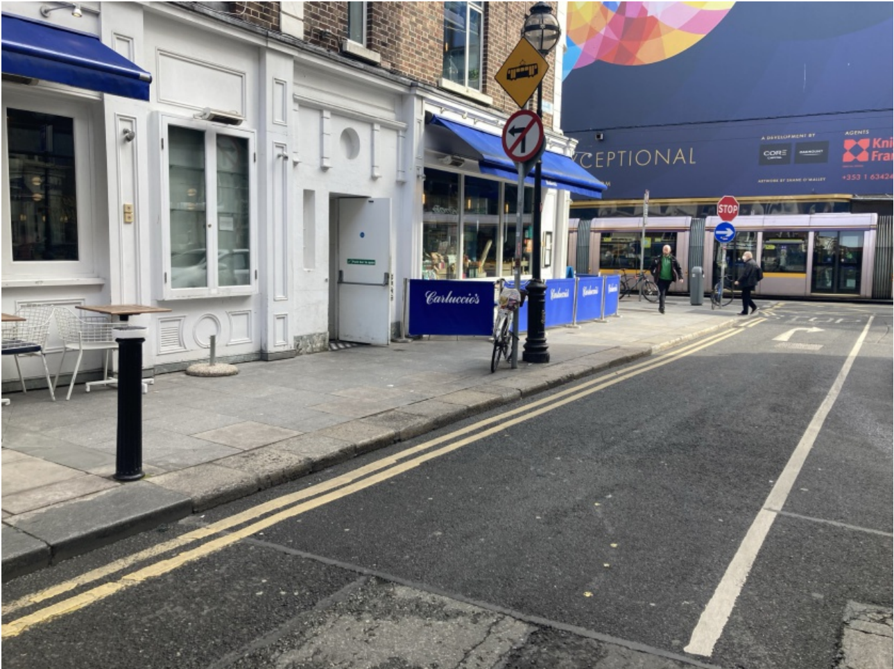
Feature Number: 10 - Integration of historical and modern granite kerbstones outside Carluccio's on Duke Street.
