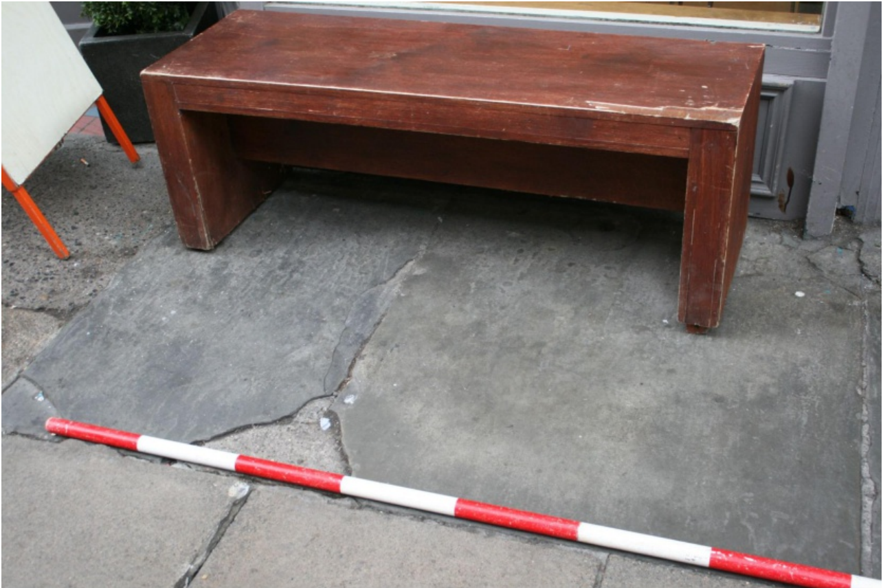
Feature Number: 43 - Flagstone entranceway, 16 Anne Street South
