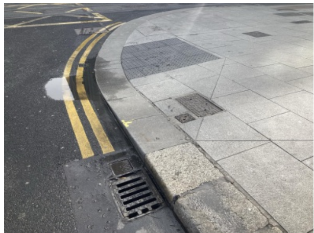
Feature Number: 11 - Transition between historical granite kerbstones and modern kerbstones on the corner of 51C Dawson Street and Duke Street.
