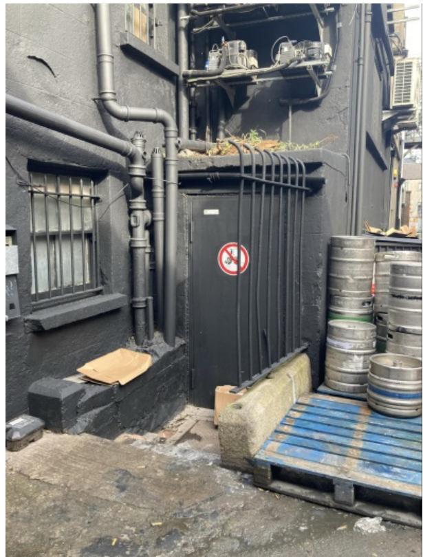
Feature Number: 65 - Entranceway at Annes Lane to 44 Grafton Street
