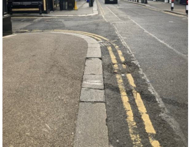
Granite kerb outside 6-7 Duke Street
