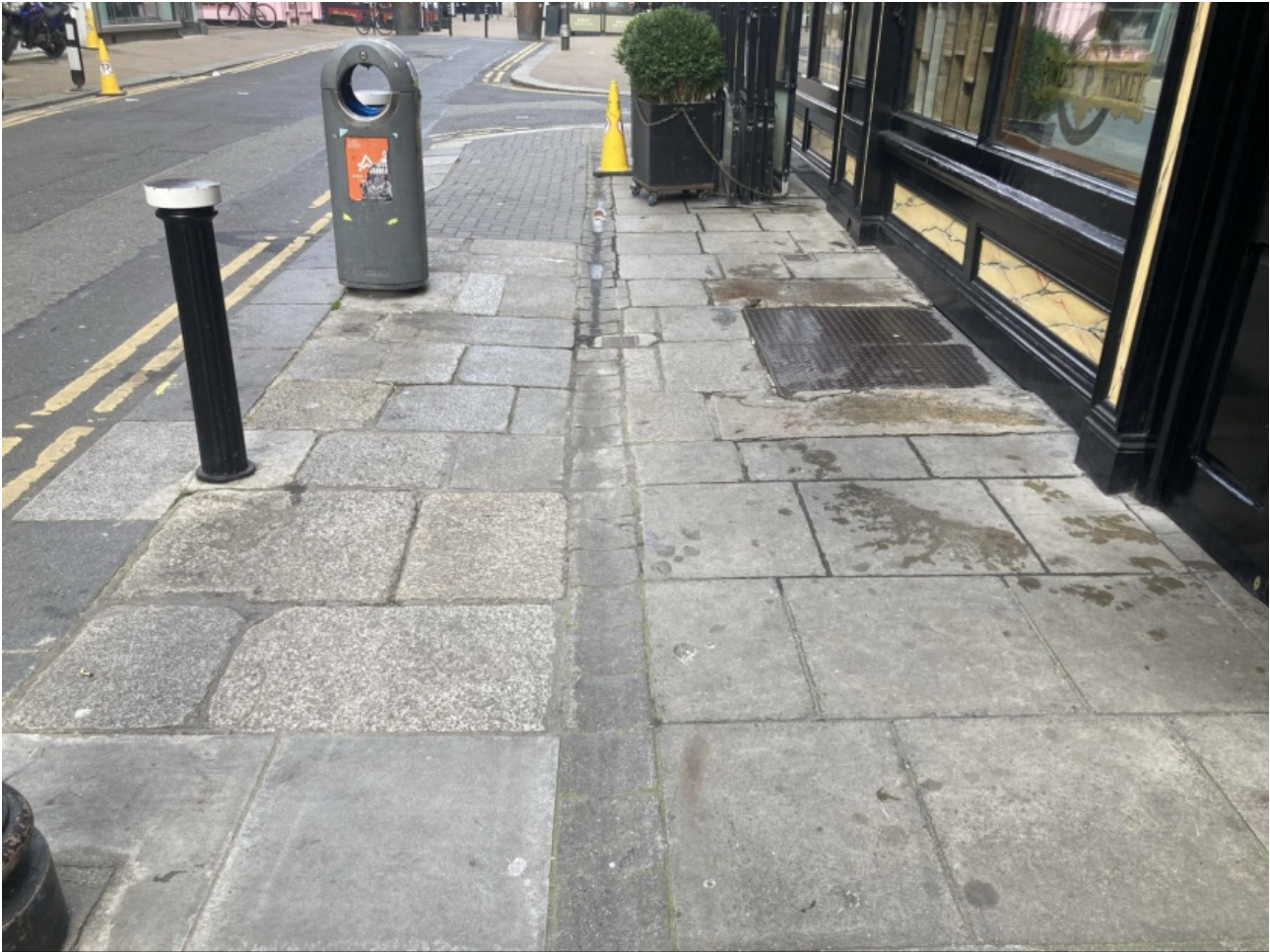
Feature Number 15: Historic granite pavement with modern inclusions and keg drop outside The Duke pub, 8-9 Duke Street
