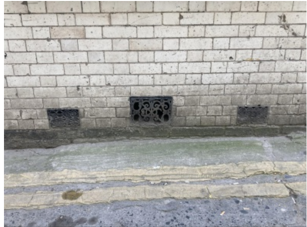
Feature 1 - Three decorative metal grates on Duke Lane (56-58 Dawson Street)
