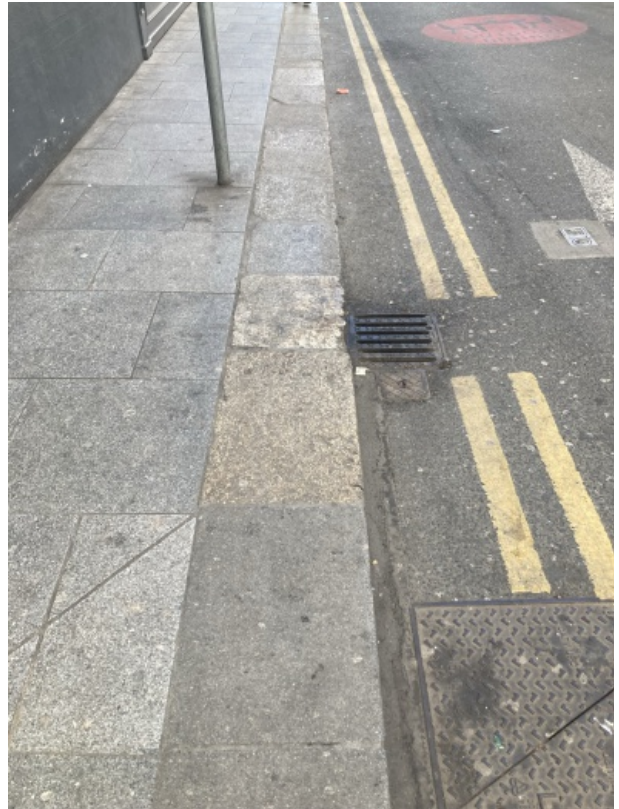
Feature Number: 33 - Granite Kerbstone - detail of join between modern and historic kerb
