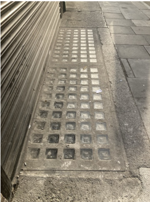
Feature Number: 59 - Lightwell, 10 Anne Street South
