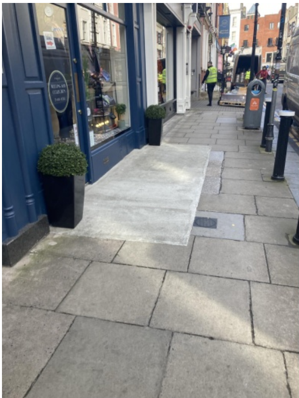
Feature Number: 14 - Survey photo from March 2022. Granite keg drop and access door now covered in concrete
