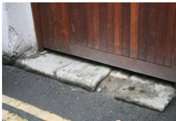
Feature Number: 63 - Granite doorstep/kerbstone, 34 Annes Lane
