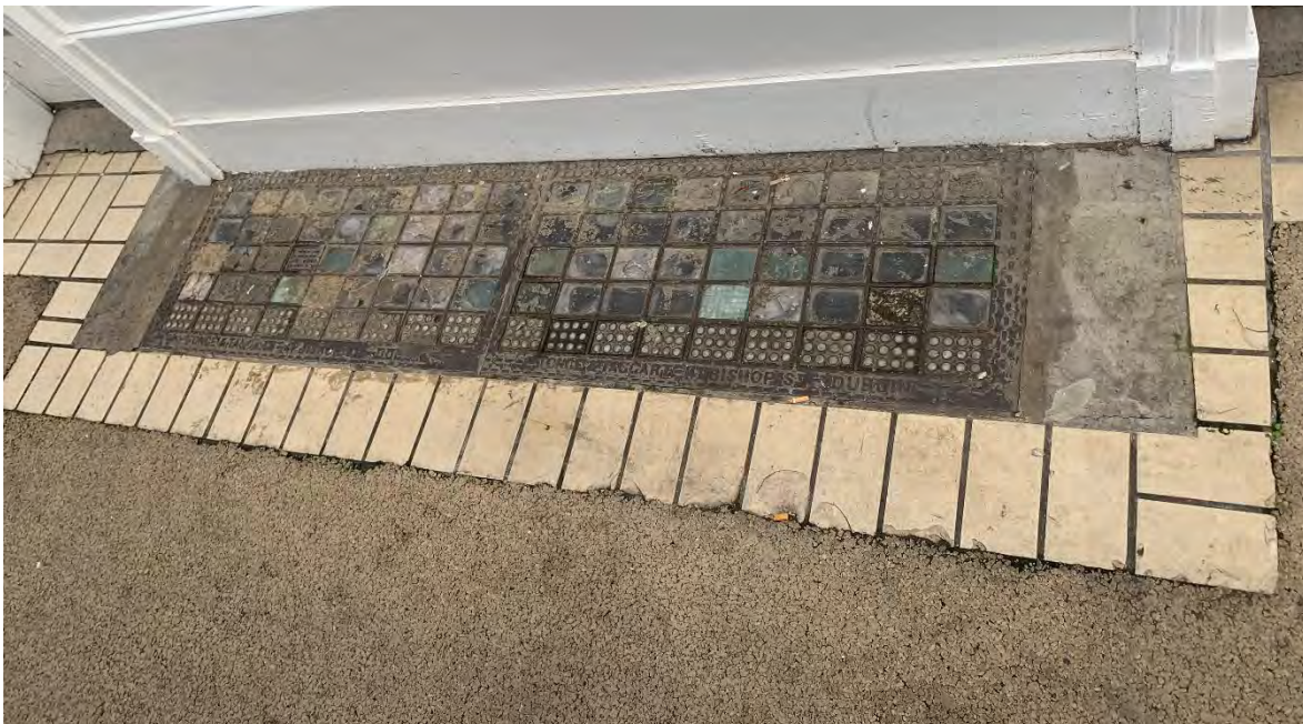
63. Photograph of historic cast iron pavement light with modern brick pavers edging, outside Smiles Dental (4 Anne St S)
