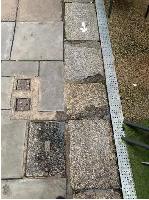
52 & 53. Photograph of example of spalled face, and chipped fronts to kerbstones outside Coffee Angel (16 Anne St S) / The Zip Yard (15 Anne St S)
