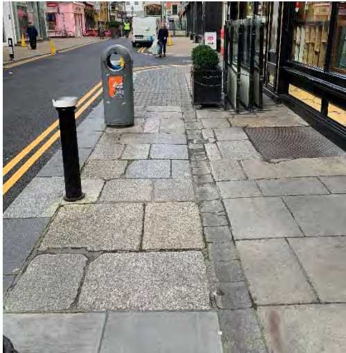
22 & 23. Photograph of section of historic Leinster granite paving to footpath outside The Duke pub (9 Duke Street), full width of footpath in places. Modern metal keg drop / cellar access may indicate position of earlier pavement light.
