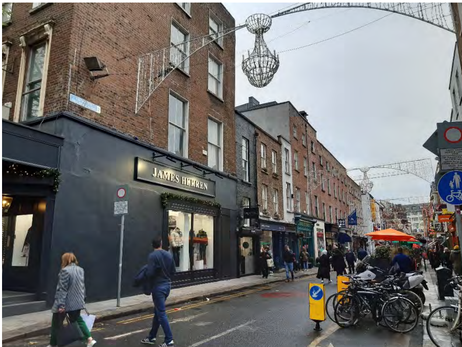
Fig 11: Streetscape photograph of southern side of Anne Street South looking west showing facade of protected structures at 18, 19, 19a, 20-26 Anne Street South
