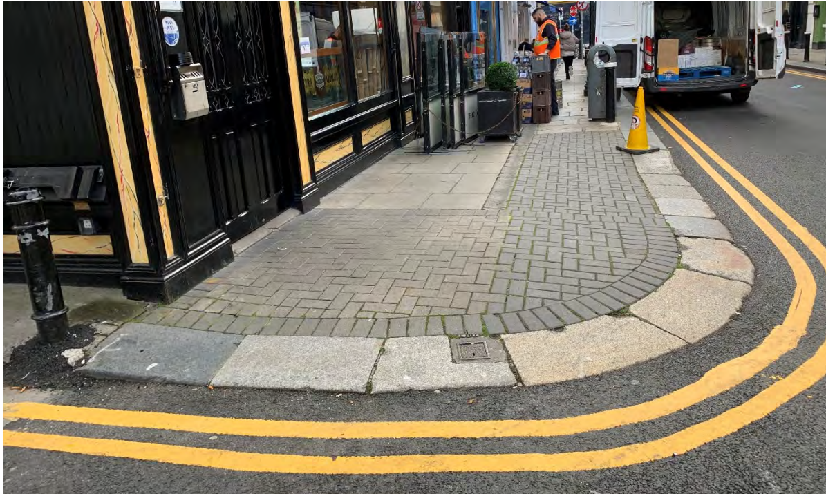
24. Photograph of historic Leinster granite kerbstones on eastern corner of Duke Street to Duke Lane. Note, there is additional conservation significance for curved historic kerbstones, which are acutely associated with their location.
