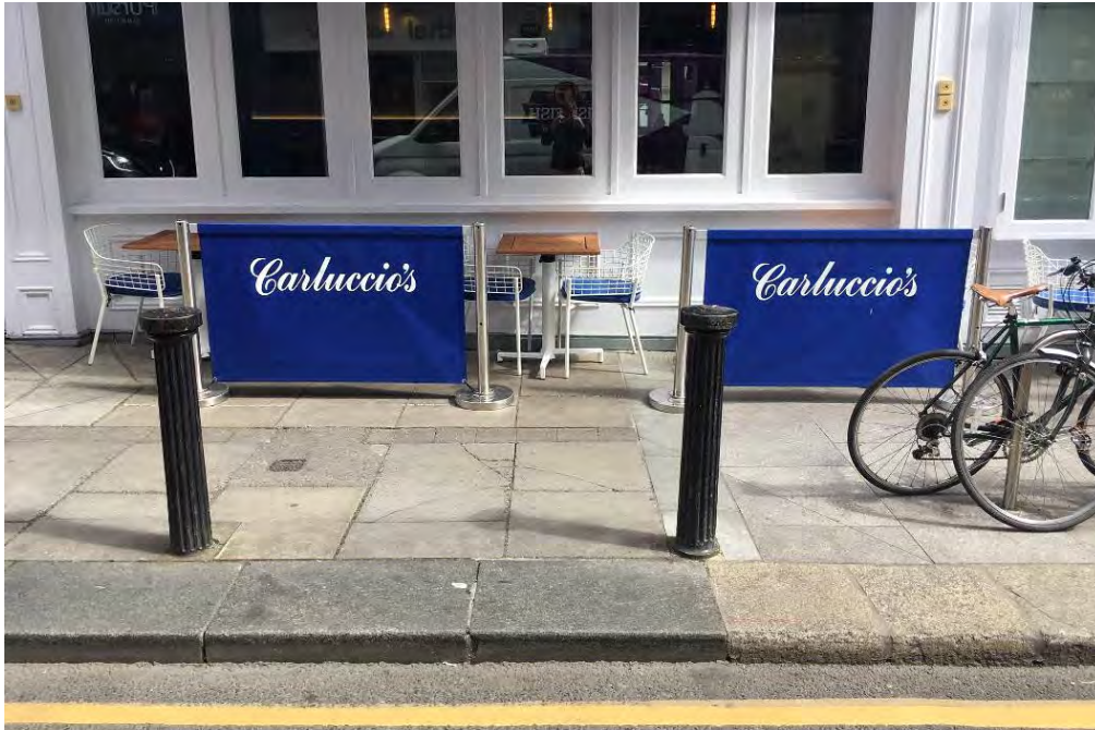
19. Photograph of modern good quality granite kerbstones to left hand side of photo outside Carluccio's with historic Leinster granite kerbstones to right hand side of photo, again outside Carluccio's (52 Dawson Street).
