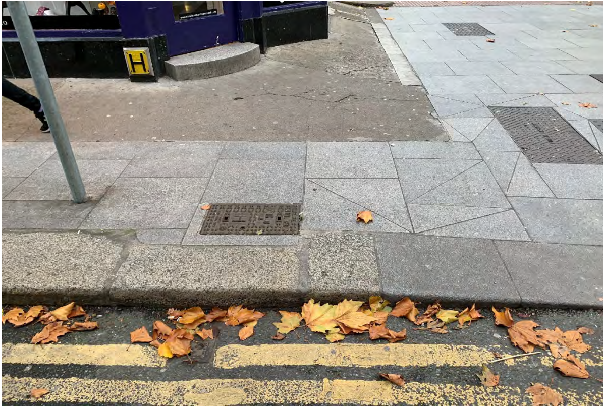
50. Photograph of slim historic Leinster Granite kerbstone that was presumably cut in the past to accommodate the nearby DCC utility cover
