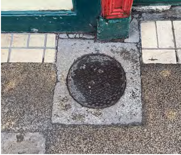
60. photograph of Historic coal hole cover set in historic Leinster Granite paver outside John Kehoe pub (9 Anne St S), and modern metal keg drop / cellar access beyond (again, may indicate previous historic cellar light).
