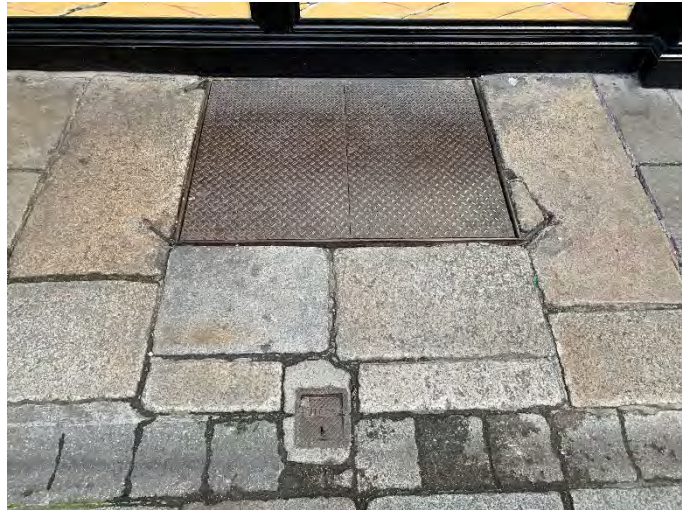
22 & 23. Photograph of section of historic Leinster granite paving to footpath outside The Duke pub (9 Duke Street), full width of footpath in places. Modern metal keg drop / cellar access may indicate position of earlier pavement light.
