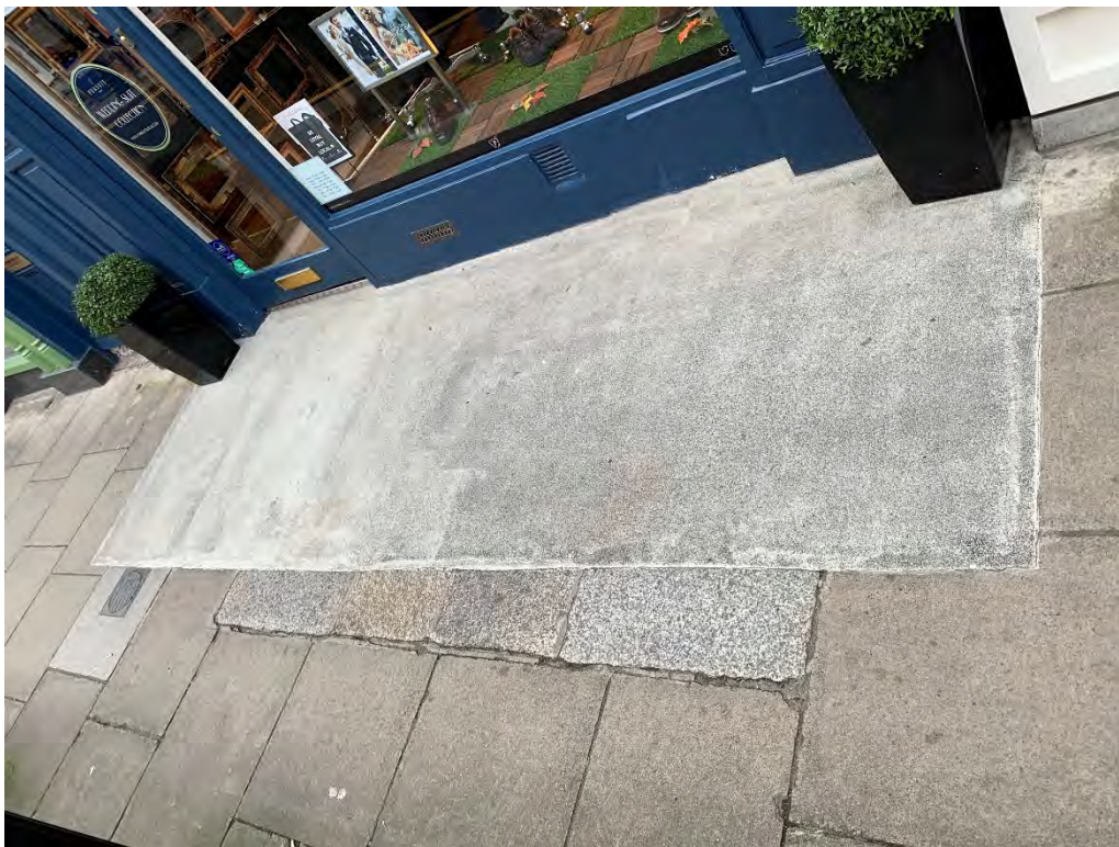
9. Photograph of former modern metal keg drop / cellar access (now filled in with concrete) outside Pursuit Dublin (14 Duke Street), with historic Leinster granite edge pavers to part.
