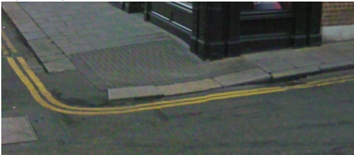
38. Photograph supplied by Phillip Dunne, Roads design department, DCC, dating from 2010 showing a larger quantity of historic Leinster Granite kerbstones at the location of photo 37 (corner of Anne Street South and Anne's Lane on eastern side). This kerb has been removed because an ESB utility cable below was stopping the proper bedding of the stone and it was repeatedly being damaged.
