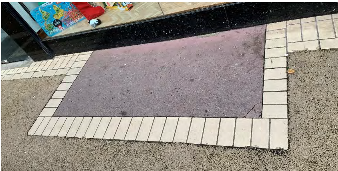
33. Photograph of infilled pavement light outside TM Lewis (32-33 Anne St S)
