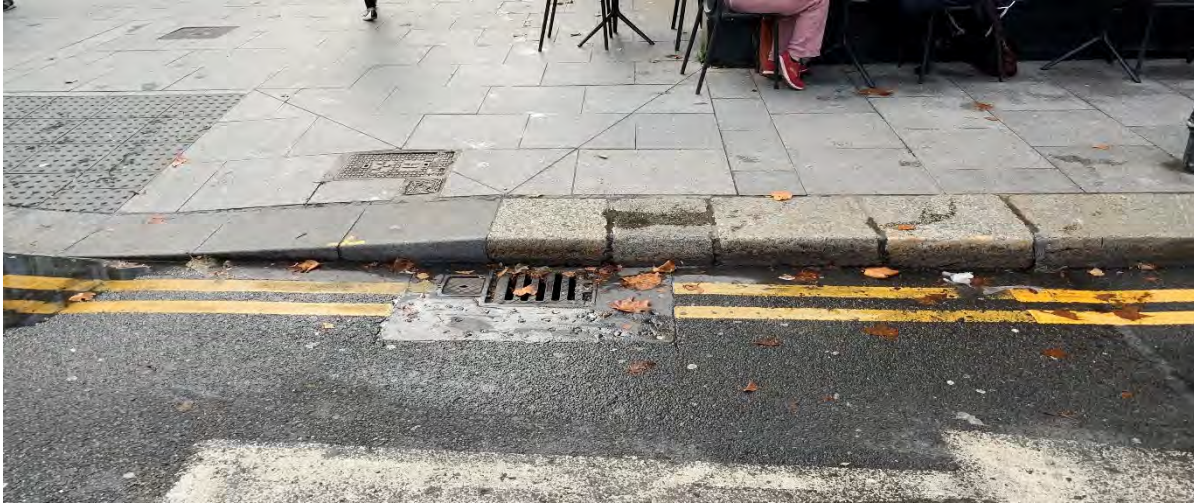
17. Photograph of historic Leinster granite kerbstones and junction with modern kerbstones at dished pedestrian crossing outside Butlers Chocolate Cafe (51c Dawson Street) / Dawson Street footpath.
