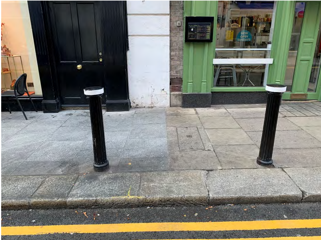
12. Photograph of historic Leinster granite kerbstones and modern granite paved footpath outside Butlers Chocolate Café (51c Dawson Street) on right hand side of photo, and more recent granite kerbstones (note finer rounded edge) and concrete pavers outside Yum Thai noodle bar (13 Duke Street) on left hand side of photo.
