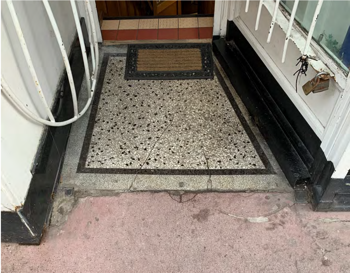
62. Photograph of terrazzo lobby to Gallery @ No Six (6 Anne St S)
