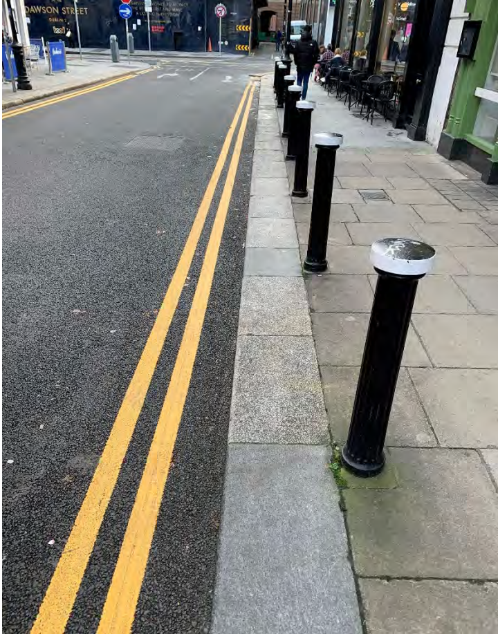
10. Photograph of modern good quality granite kerbstones outside Bang and Olufsen and Pursuit Dublin (14-15 Duke Street)
