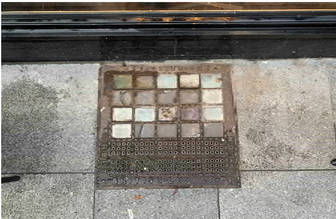
13. Photograph of historic cast iron pavement light with no edging band, set within modern granite paving, outside Butlers Chocolate Café (51c Dawson Street).
