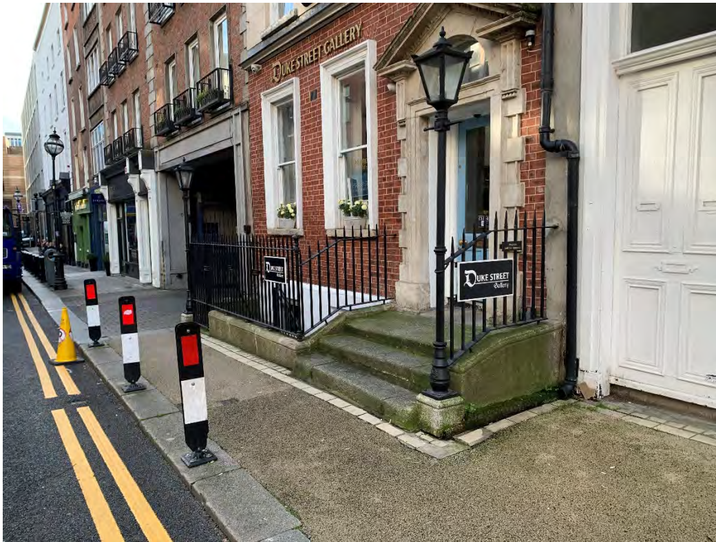
7. Photograph of private landing outside Duke Street Gallery (17 Duke Street) with historic Leinster granite steps and low wall and cast iron railing above.
