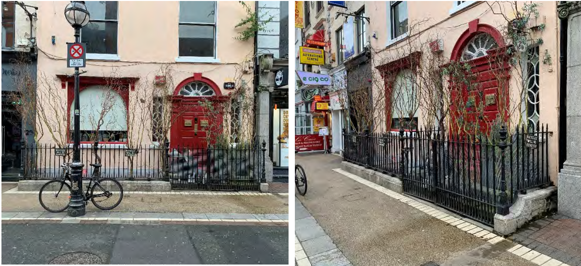
34 & 35. Photograph of private landing outside Brendan Joseph Store & Design Studio (30 Anne St S) with historic Leinster granite steps and low wall and cast iron railing above.
