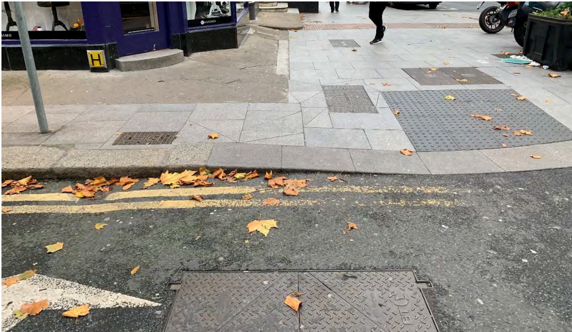
49. Photograph of historic Leinster granite kerbstones and junction with modern kerbstones at dished pedestrian crossing outside Massimo (45 Dawson Street) / Dawson Street footpath
