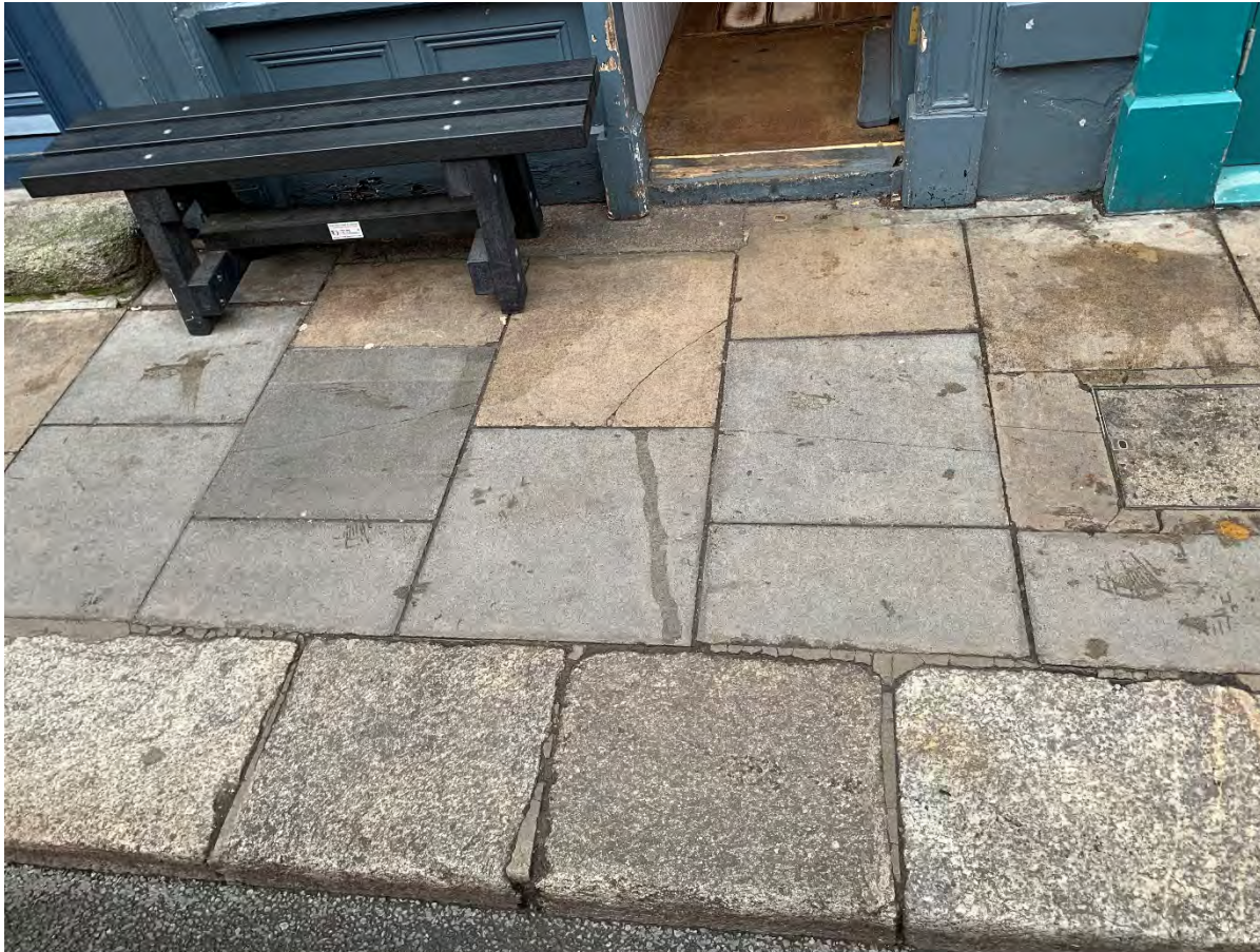
44. Photograph of historic Leinster granite section just in front of shopfront to Dublin Barista School (19 Anne St S)
