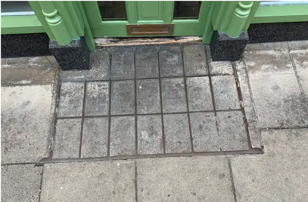
11. Photograph of historic cast iron cellar pavement light infilled with concrete outside Yum Thai noodle bar. (13 Duke Street)
