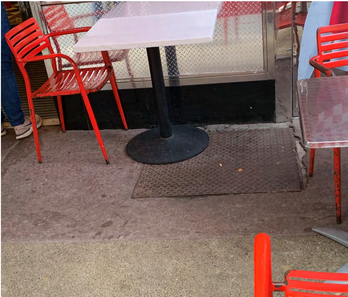
61. Photograph of modern metal keg drop / cellar access outside Eddie Rockets (7 Anne St S) – may indicate previous historic cellar light
