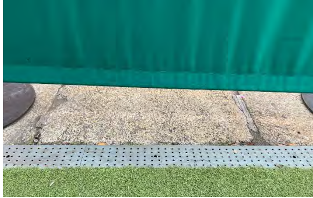
52 & 53. Photograph of example of spalled face, and chipped fronts to kerbstones outside Coffee Angel (16 Anne St S) / The Zip Yard (15 Anne St S)
