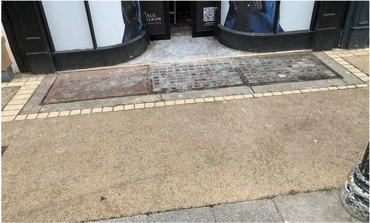
64. Photograph of historic cast iron pavement light with historic granite edging, outside Inglot (10 Anne St S)
