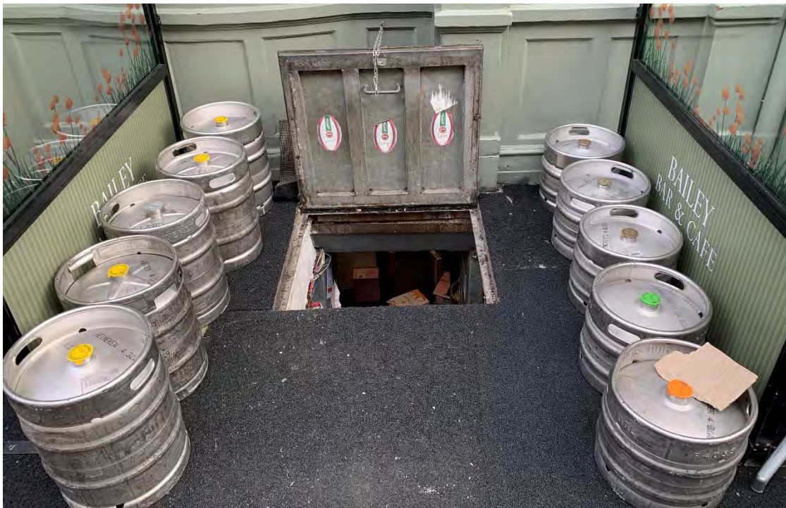
27. Photograph of modern metal keg-drop / cellar cover outside the Bailey (1-4 Duke Street). Note, on the day of survey it was not possible to survey footpath materials under the outdoor dining area outside the Bailey, as ground coverings were in place. It is noted from previous site inspections that a small section of Historic Leinster Granite edge paving is located at the modern keg-drop, however the full extent of the ground materials have not been able to be surveyed.
