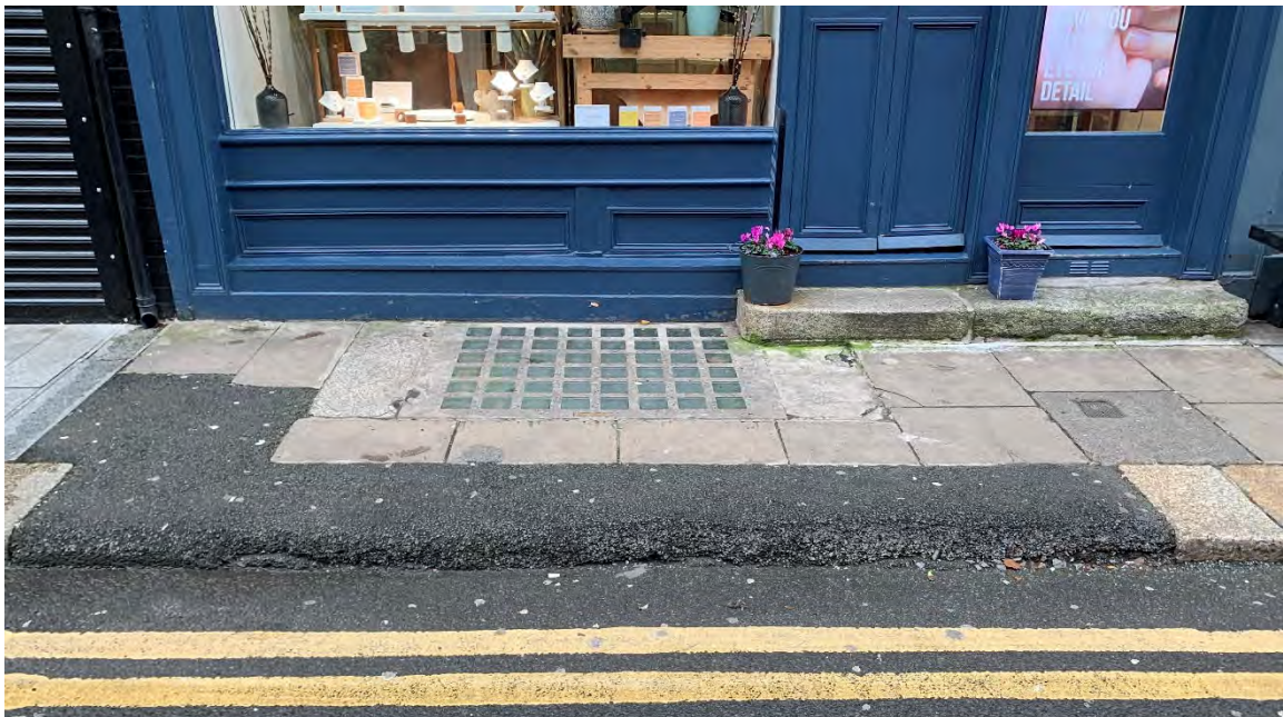
45. Photograph of modern concrete pavement light with 1no historic Leinster granite edge paver (to left), and some historic Leinster granite kerbstones to either side of large asphalt repair, outside Deirdre O Donnell jeweller (19 Anne St S).
