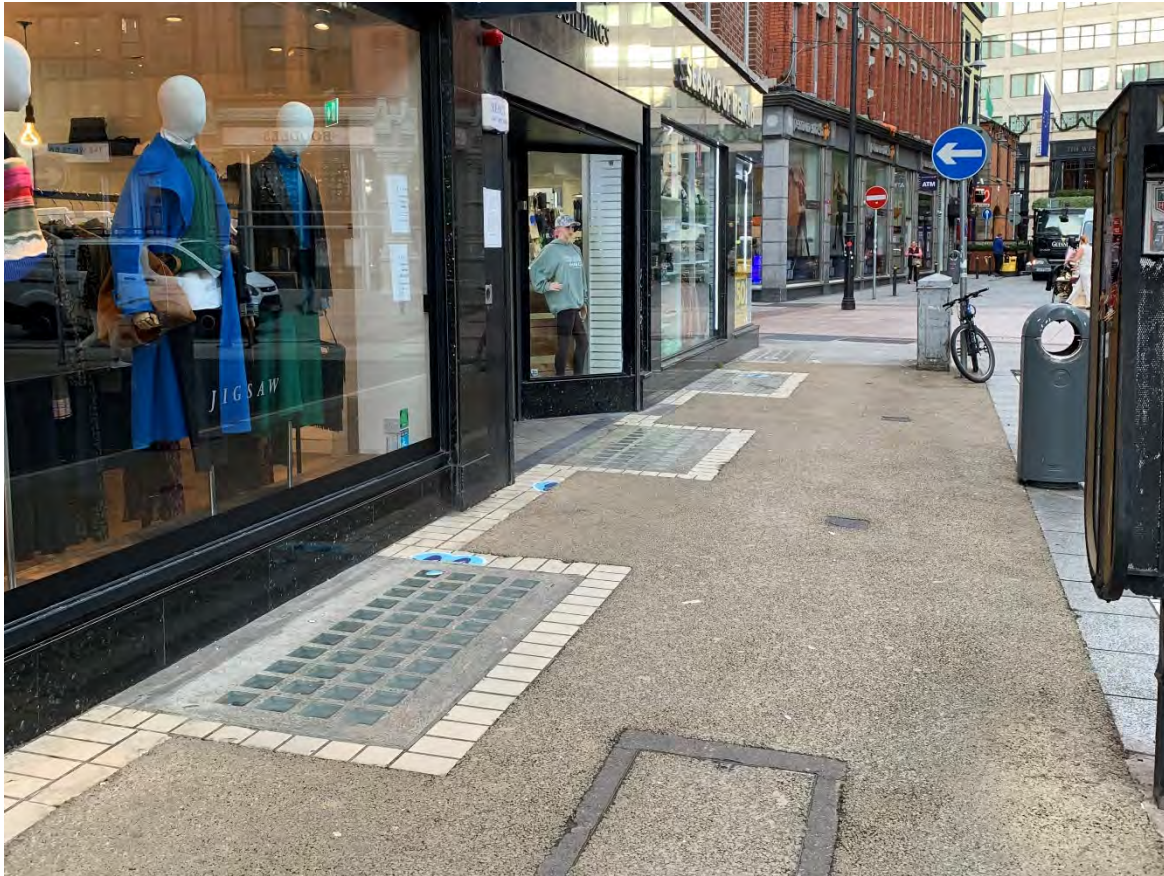
32. Photograph of modern concrete pavement lights set within 1980's Grafton street materials, Seasons of Ireland, Jigsaw (34 Anne St S) and TM Lewin (32-33 Anne St S) : 5no – note 1no furthest east infilled, concrete.
