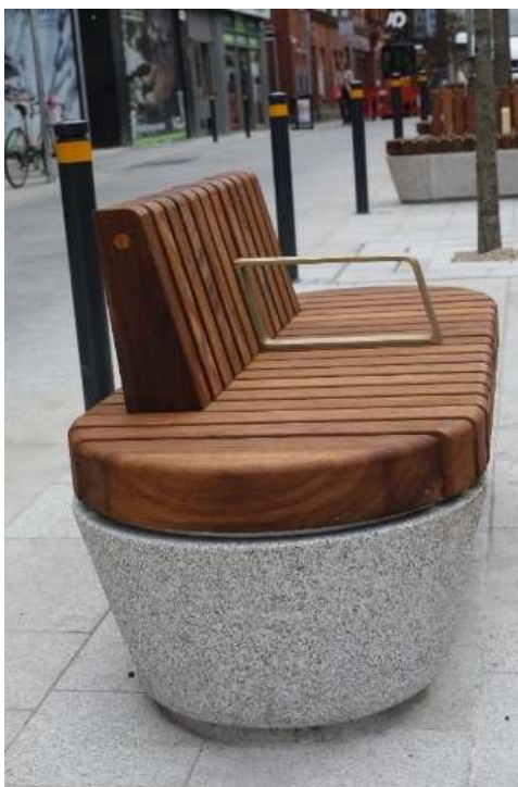
Fig 10: Image of bench on Chatham Street with Leinster granite base, timber seat and backrest and metal arm rest
