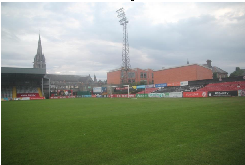
Plate 3 Looking to the southwest of site, Des Kelly Stand to the right of plate.
