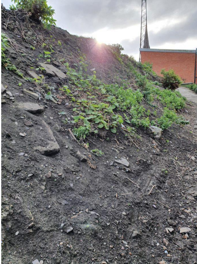
Photo 17: Berm where Des Kelly Stands used to be located
