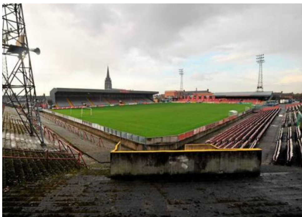
Figure 4 - View from the Northeast corner of the Connaught Street Stand (Source IDOM).
