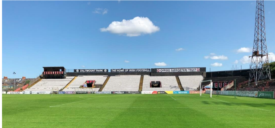
Photograph 2: Connaught Avenue Stand prior to demolition
