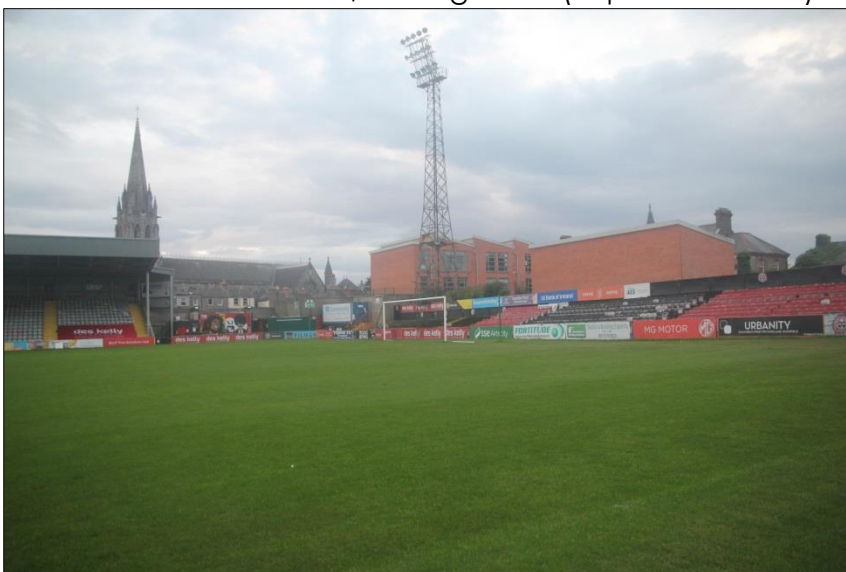
Plate 3 Looking to the southwest of site, Des Kelly Stand to the right of plate.
