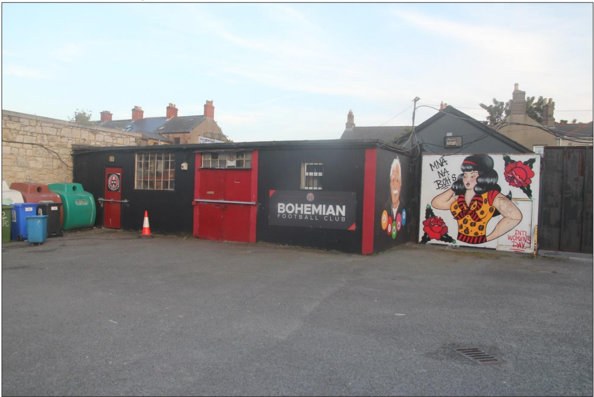
Plate 13 Buildings onsite, Negligible bat roost potential.
