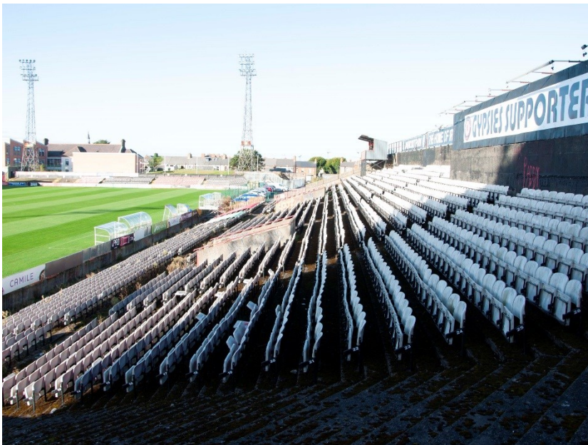
Plate 3: Connaught St. Stand, along the north, facing west.
