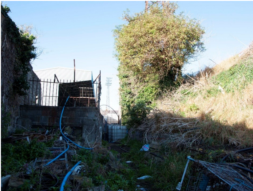
Plate 19: View behind Tramway Stand showing earthen embankment construction, facing south.
