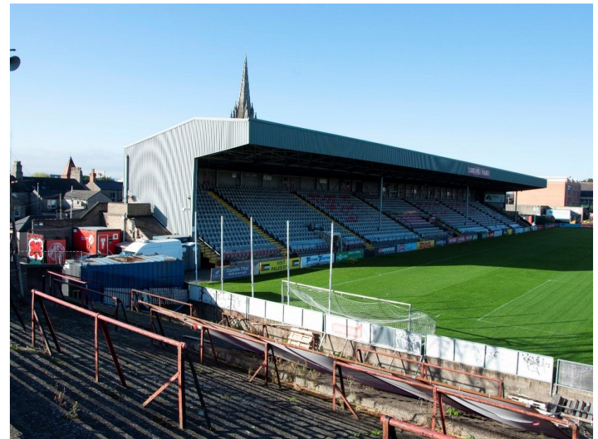
Plate 4: Jodi Stand, view from Tramway End Stand, facing southwest.
