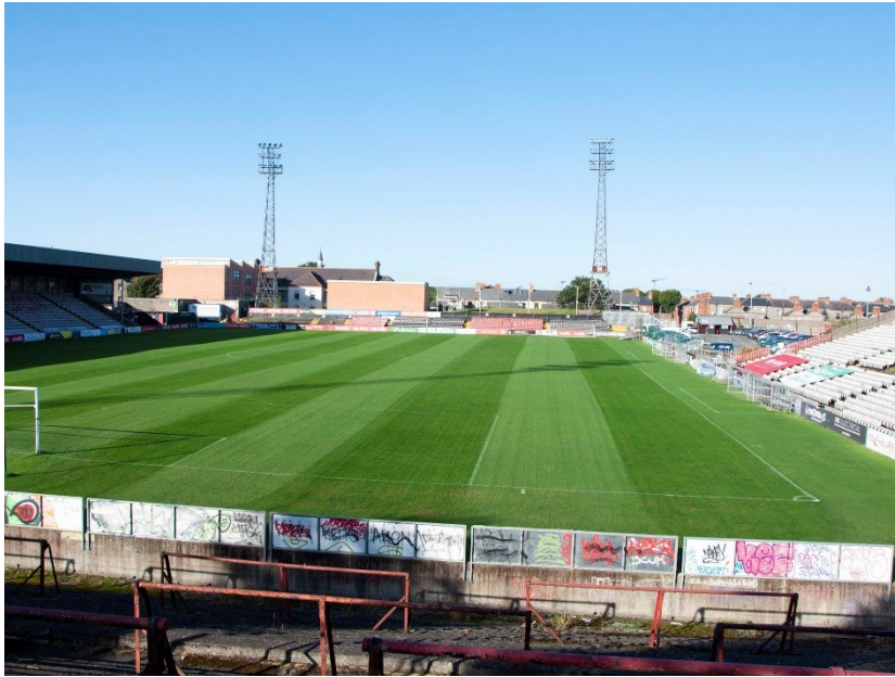
Plate 1: Site overview from Tramway End Stand, facing west.
