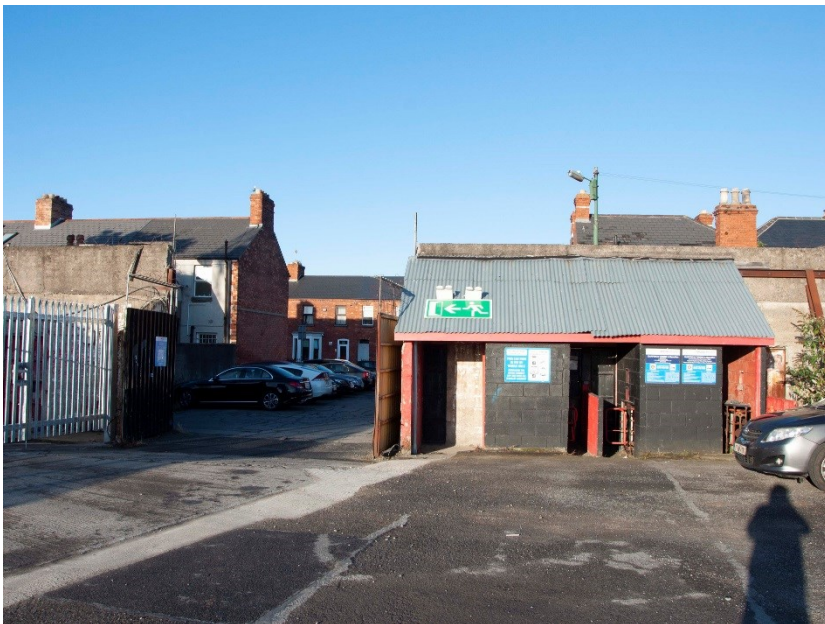
Plate 11: Entrance off St Peters Rd., view from the carpark, facing west.
