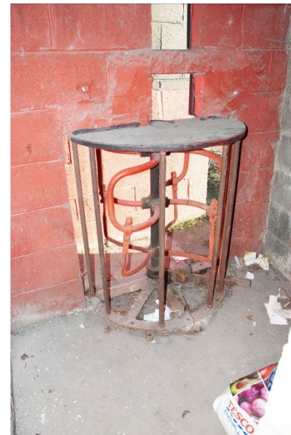
Plate 16: 1920s/1930s cast iron 'rush preventive' turnstile.
