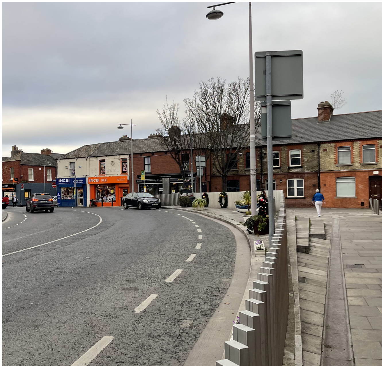
ABOVE: The existing super elevated road bend along the R802 Bridge Street.
