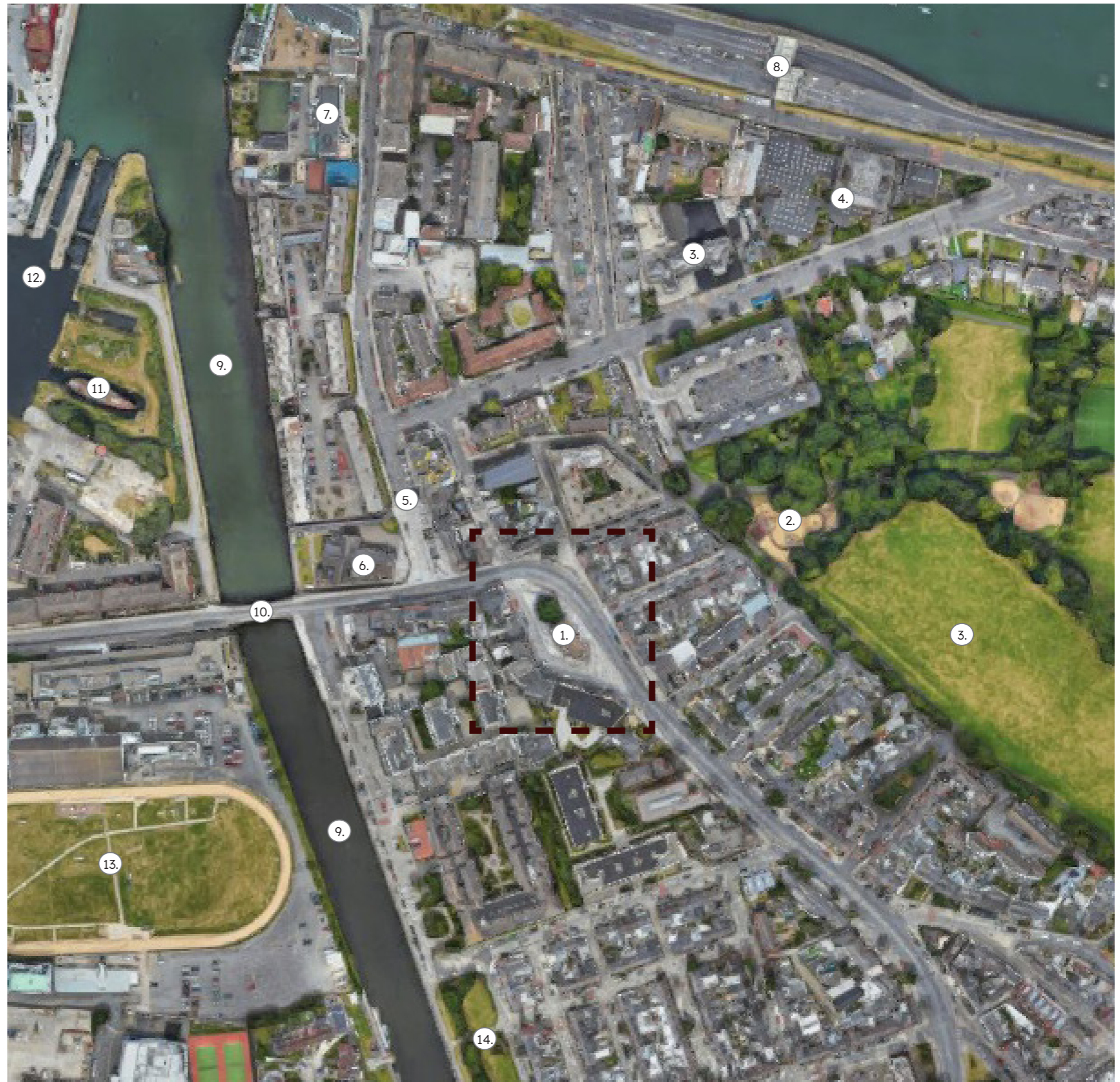
Aerial Image highlighting the application site (red) and the surrounding context . For illustrative purposes only.
