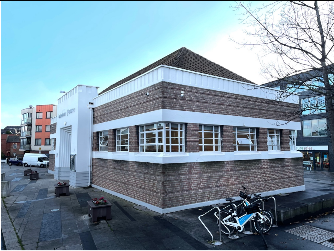
3. - Oblique view taken from the North East
