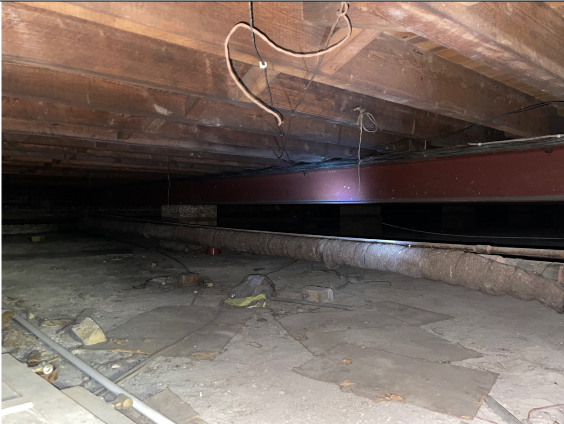
36 - View of subfloor crawlspace void beneath main library
