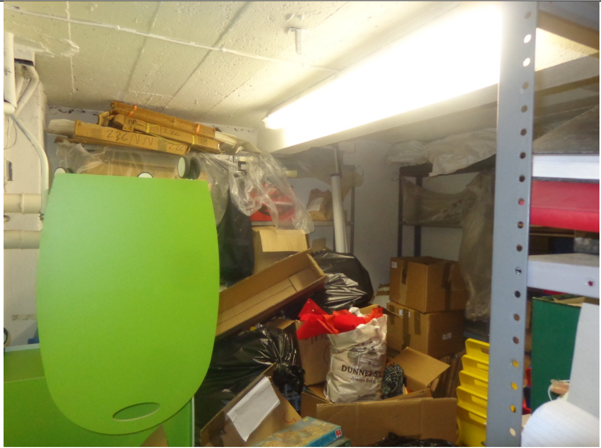
43- View of concrete ceiling / floor above small basement store
