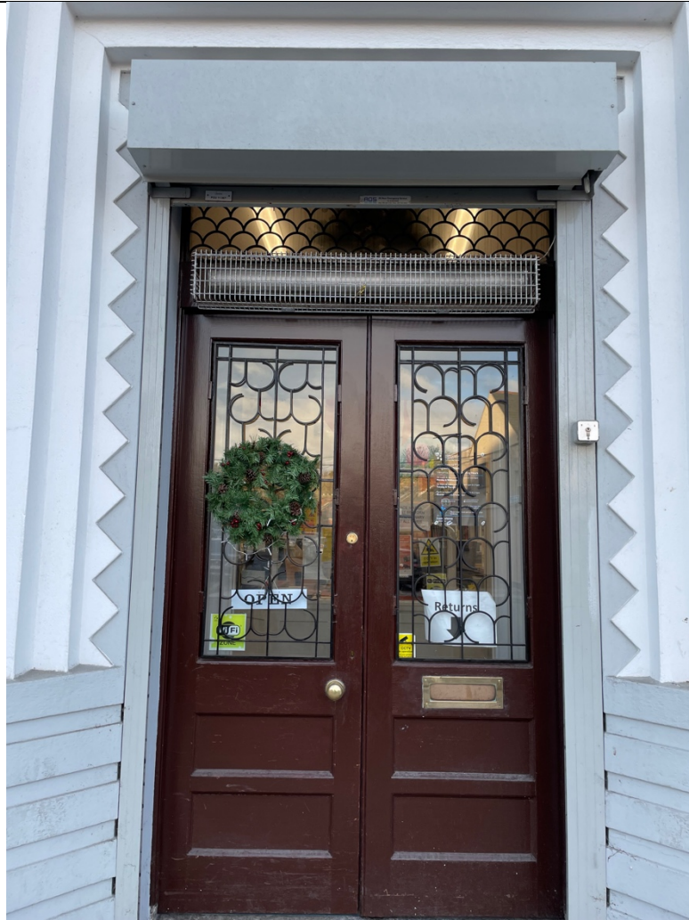
5. – Front entrance door detail
