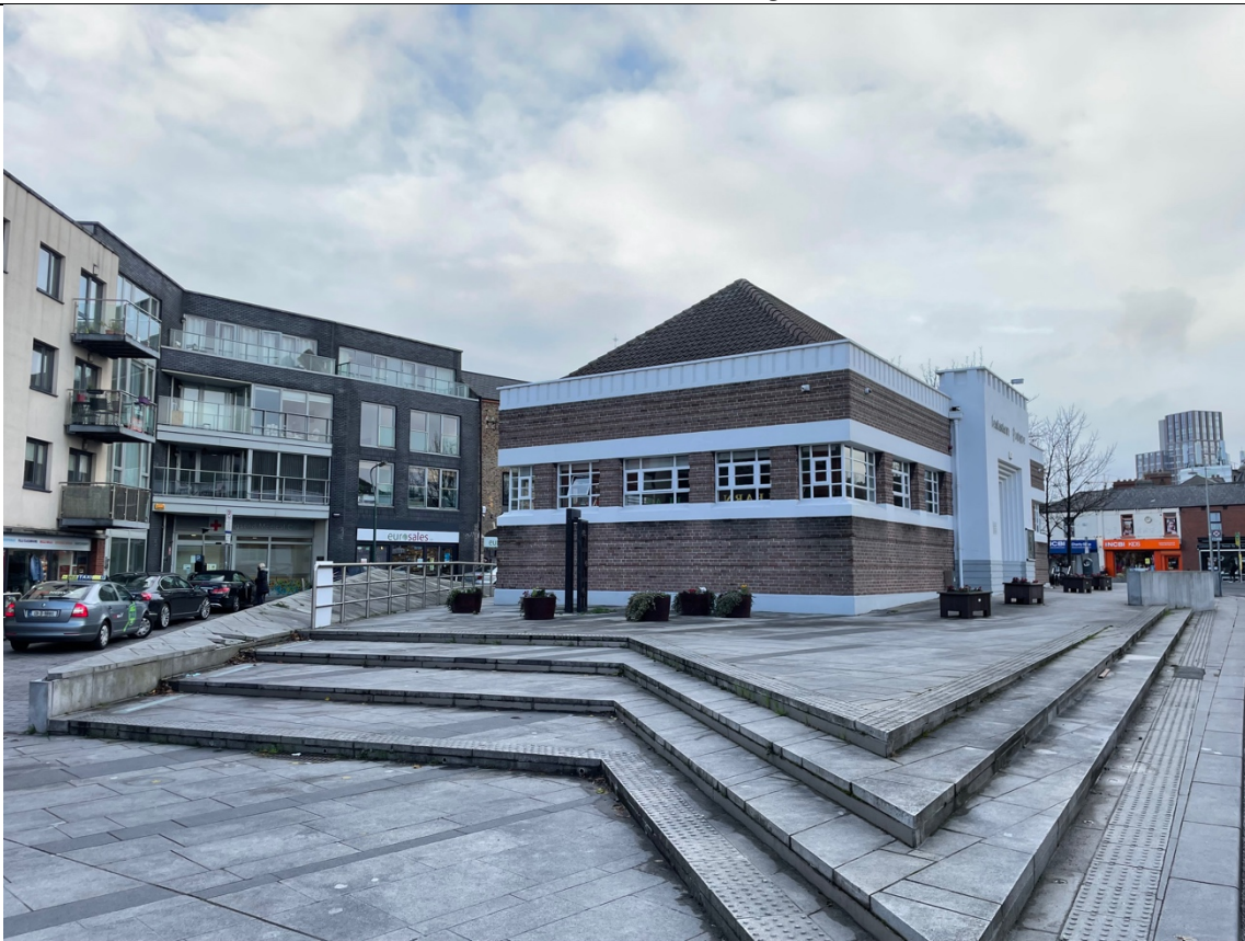
2. - Oblique view taken from the South East
