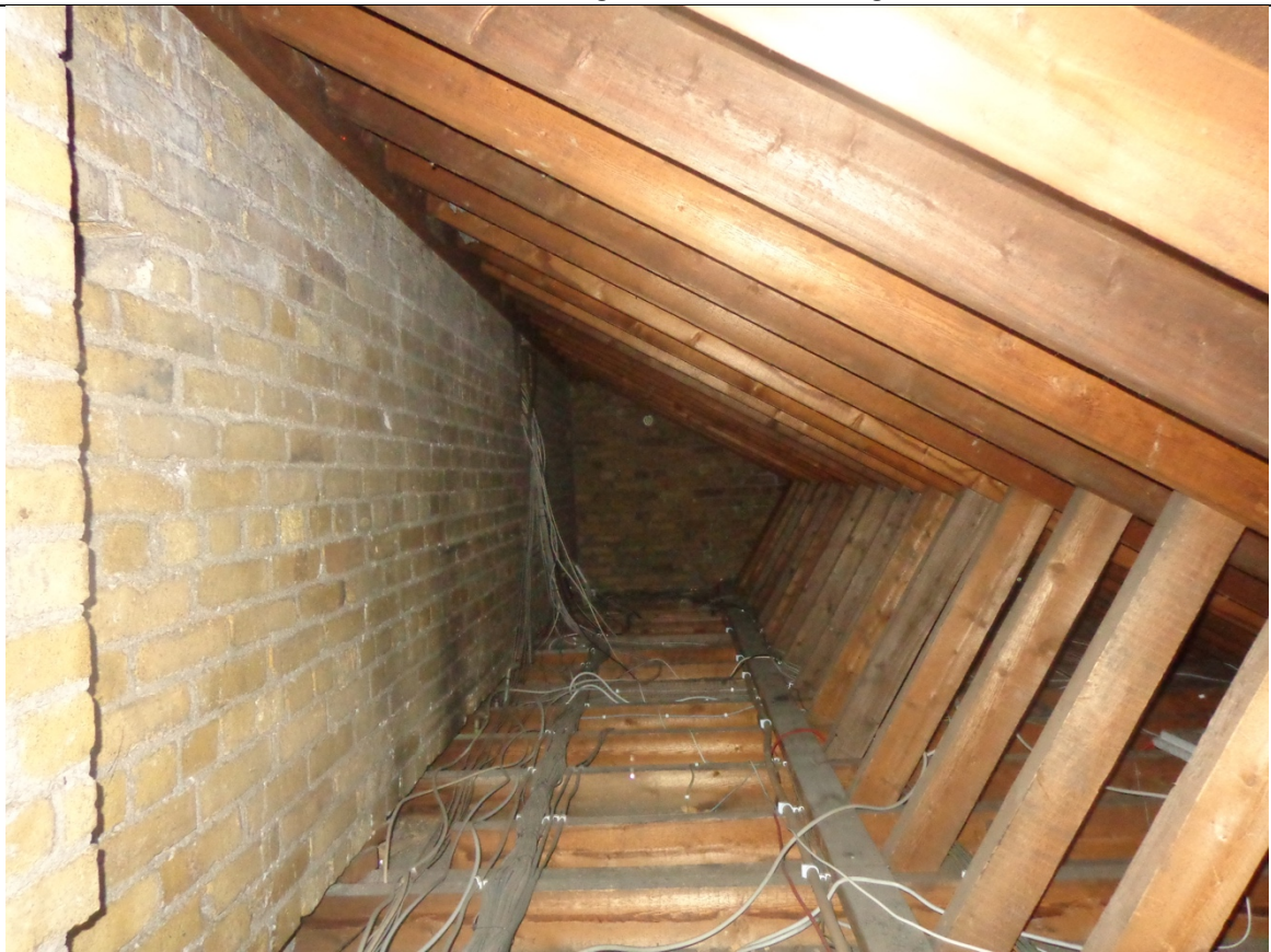
34- View of roof void over rear lean-to
