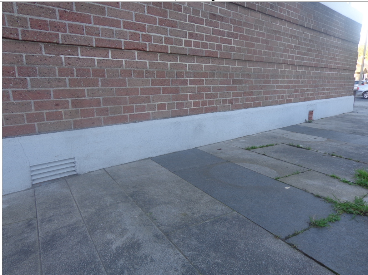
12. View of subfloor wall vents (South wall).
