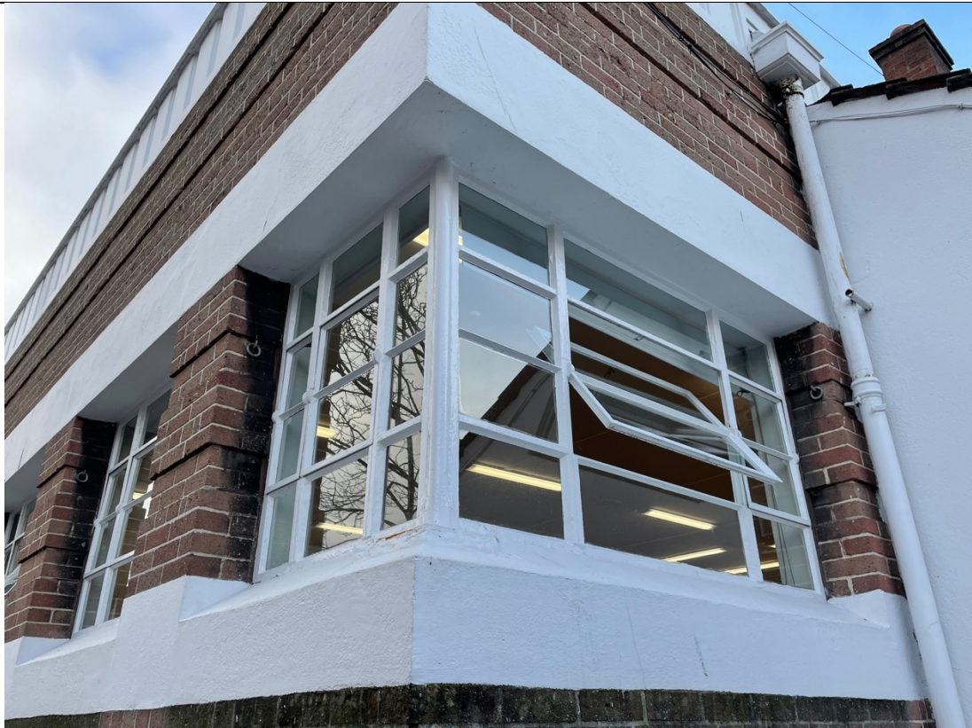
14. View of original metal Crittal window to corner
