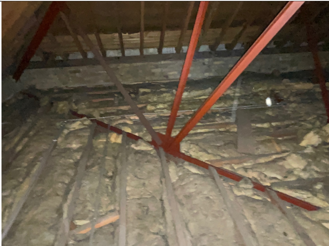
52 – View of main attic, triangulation of roof at hip trusses
