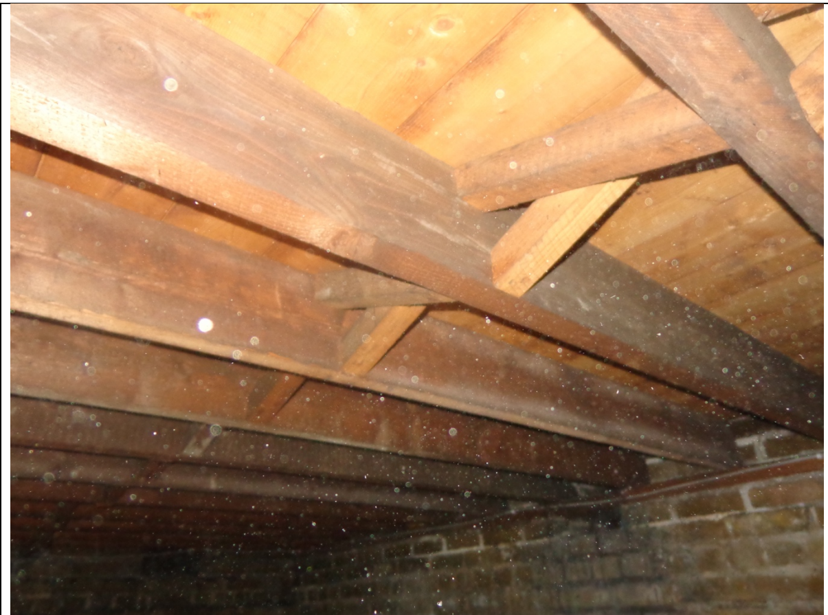
39 - View of herringbone bridging / strutting
