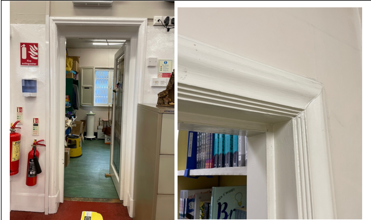
32 – Detail of original profiled architrave door joinery
