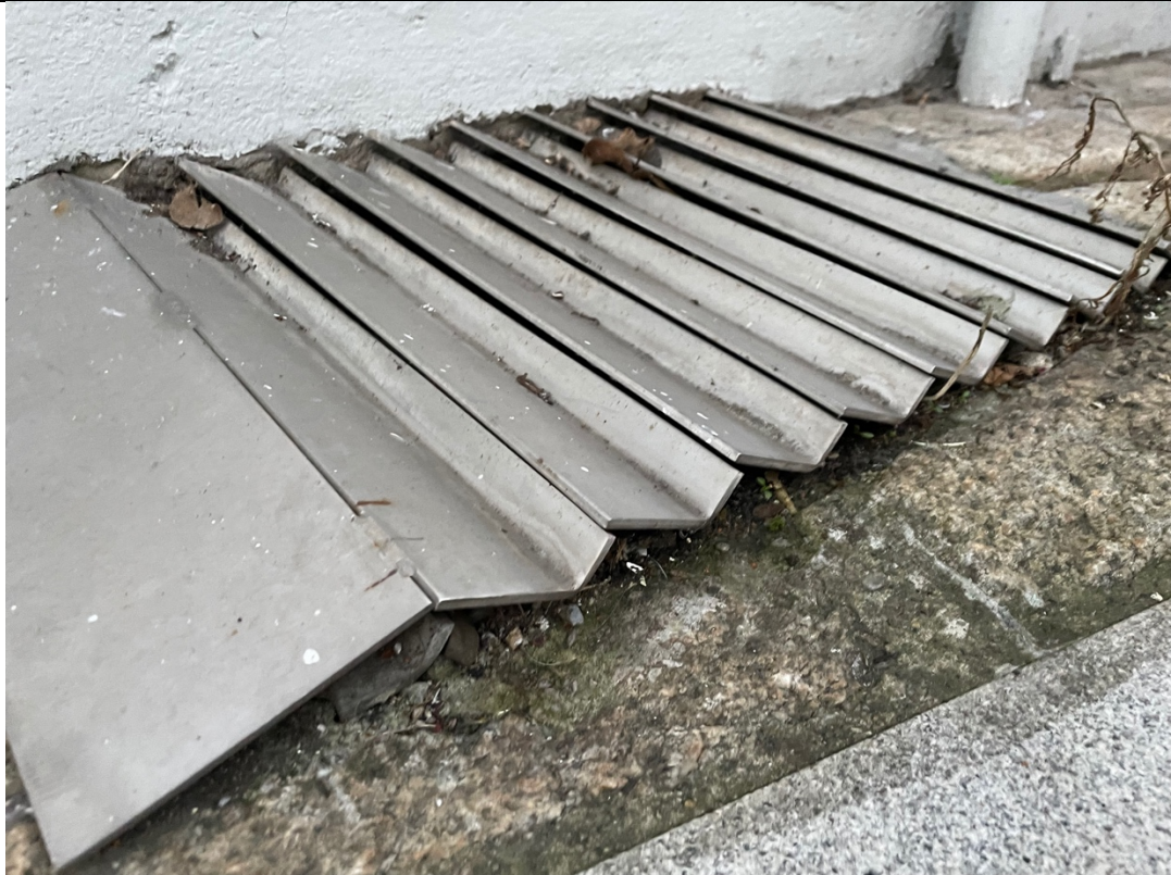
13. - View of bespoke surface vent to altered original subfloor vent locations
