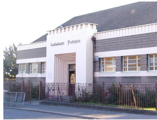
Ringsend Library (prior to 2003 works)
