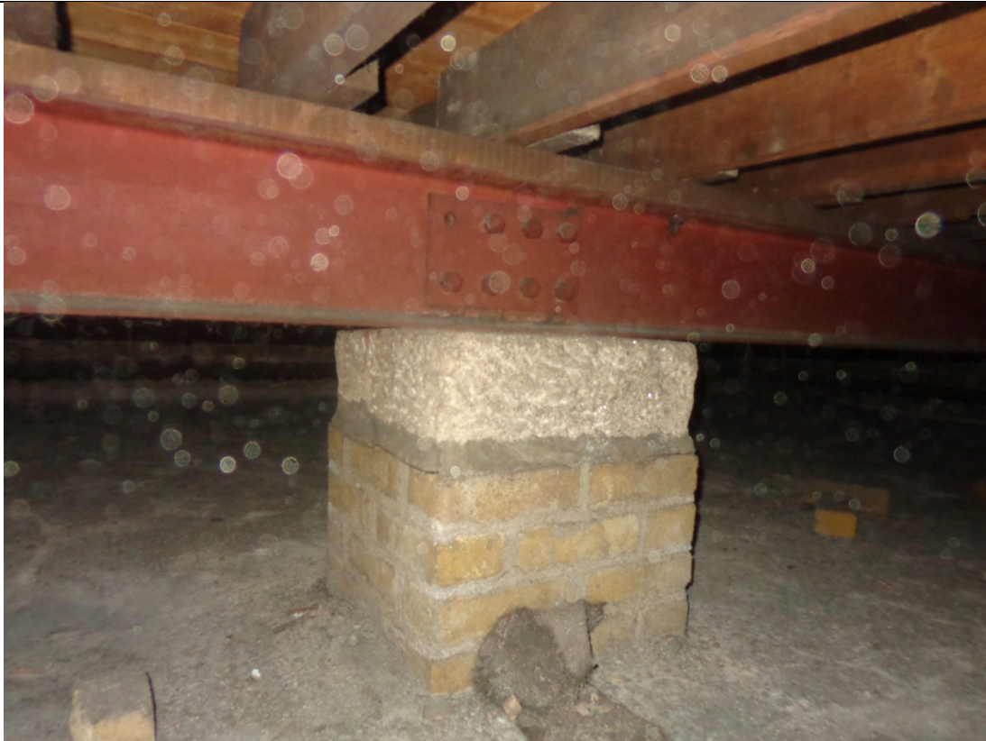
37 - View of 470 mm square brickwork tassel pier and granite padstone
