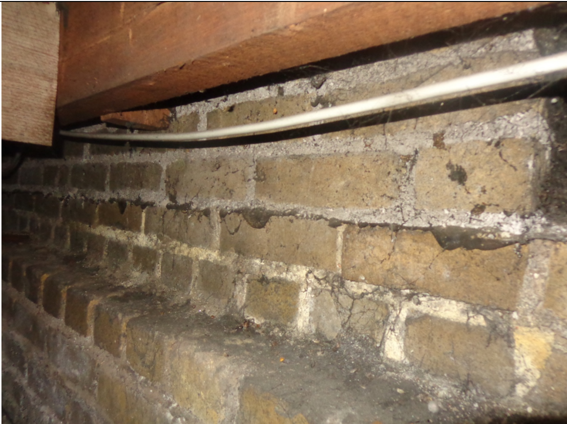
42 - View of bitumen damp proof course, viewed from within subfloor crawlspace
