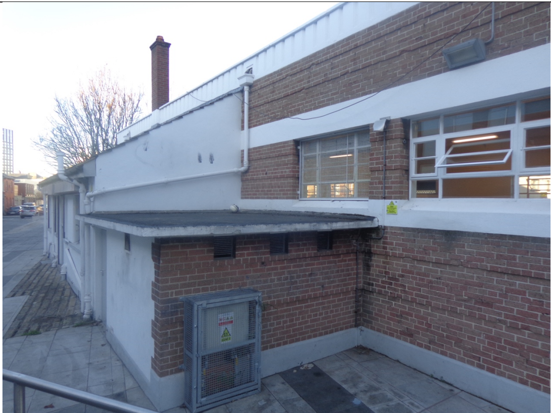
8. - View of rear plant roof and concrete flat roof over
