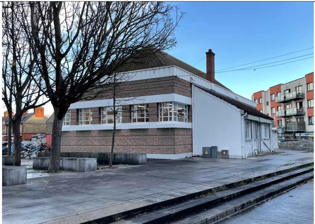
4. - Oblique view taken from the North West
