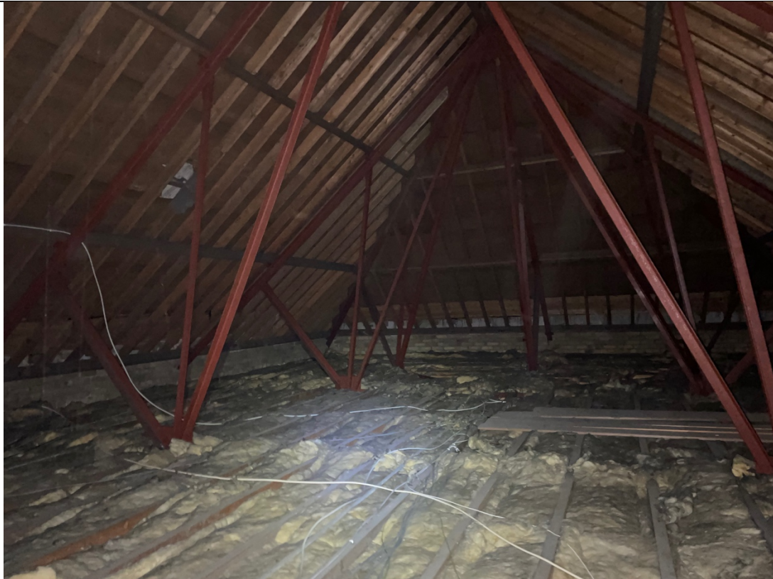
51 – View of main attic
