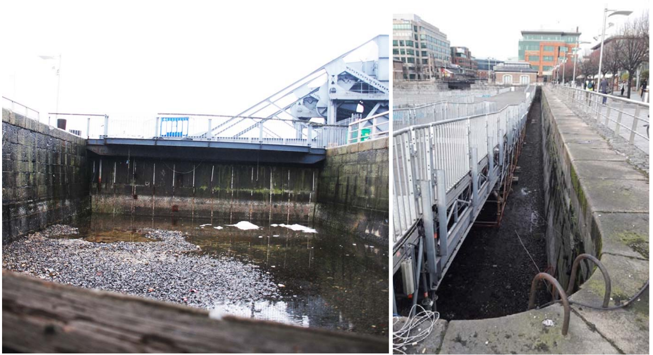
Plate 2. Poured Concrete Wall between the dock and River Liffey (left). Eastern wall, dry gravel and platform in Georges Dock (right).
