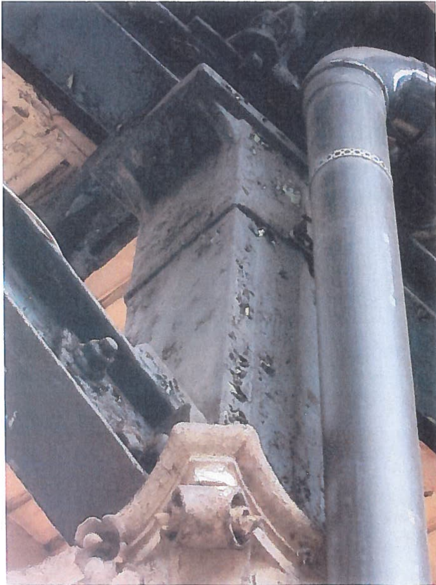
Fig 75 Rainwater pipe from roof valley positioned alongside column
