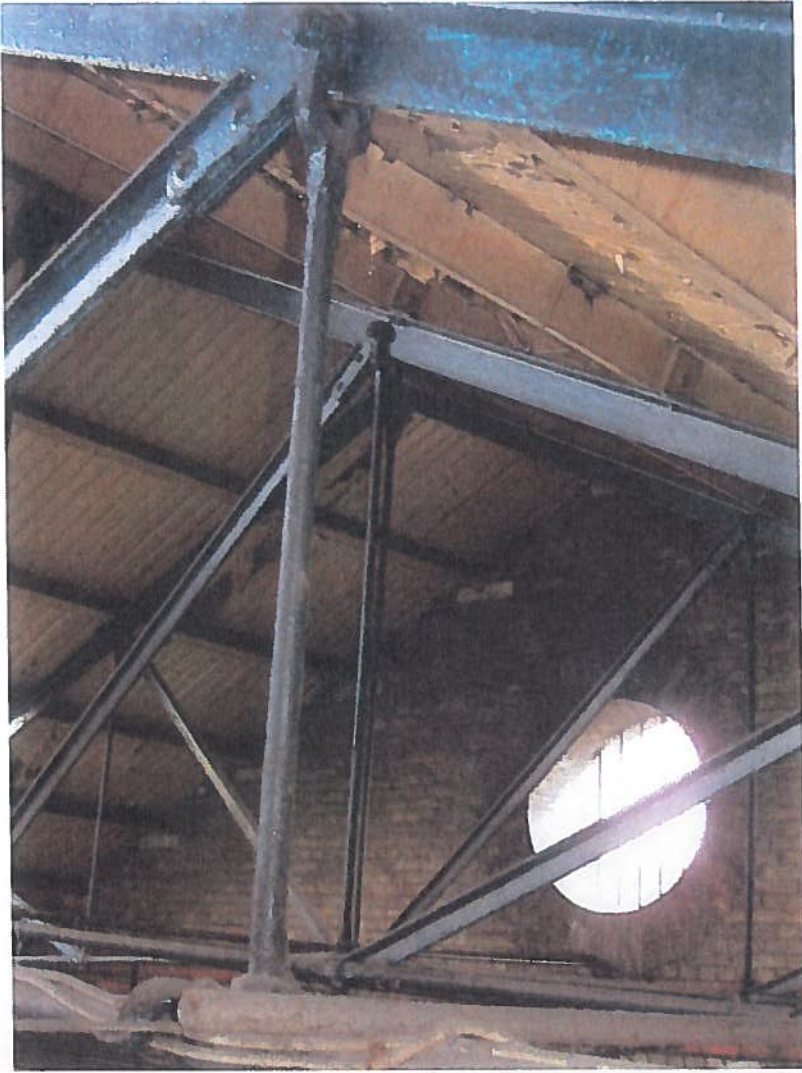
Fig 73 Ties bolted to roof trusses
