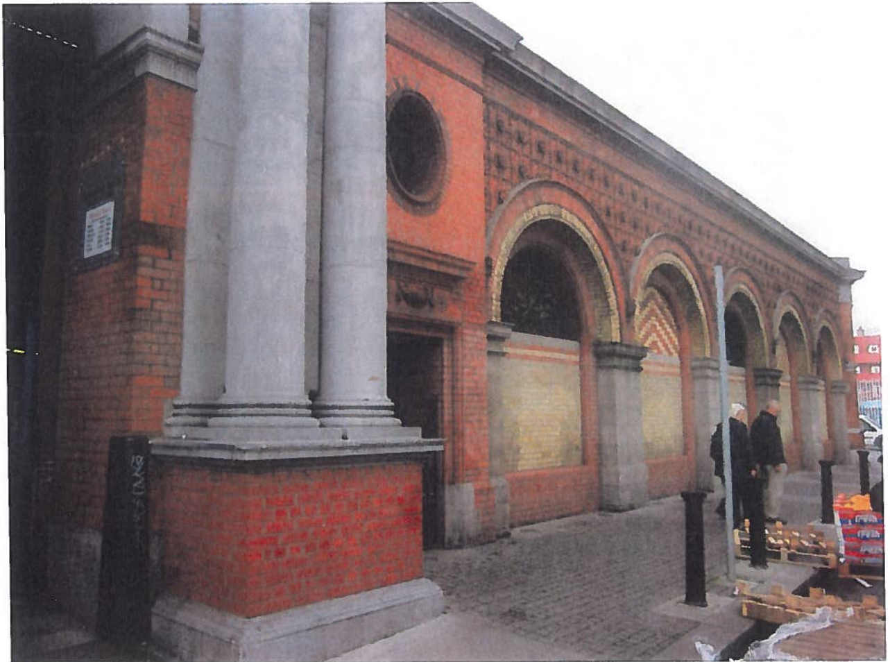
Fig 32 'On either side of these entrances are six granite piers, standing on a chamfered base and finishing on top with a moulded cap, from which spring semi-circular arches of moulded red and yellow brick, finishing with a hollow chamfered hood-moulding.'
