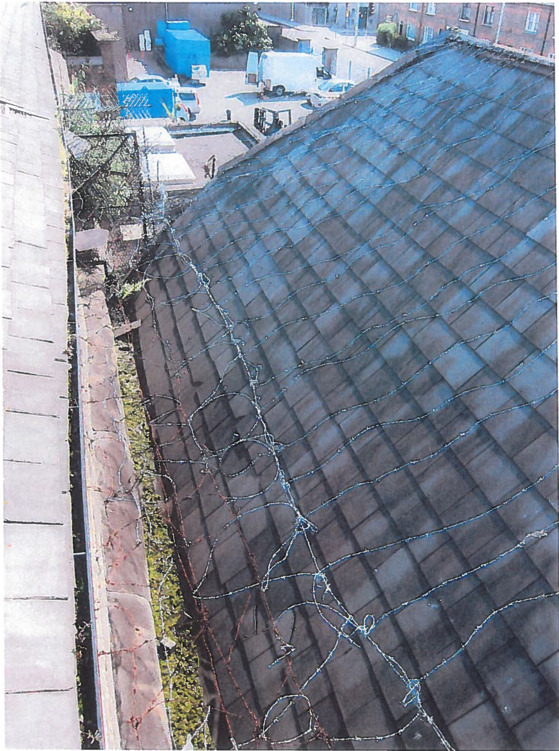
Fig 88 Roof of adjoining shop
