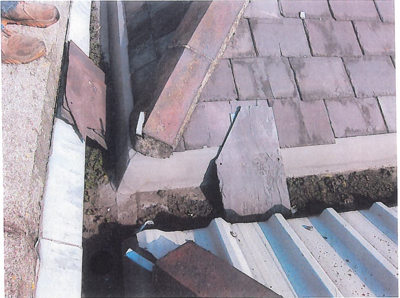
Fig 80 Parapet gutters on main elevations
