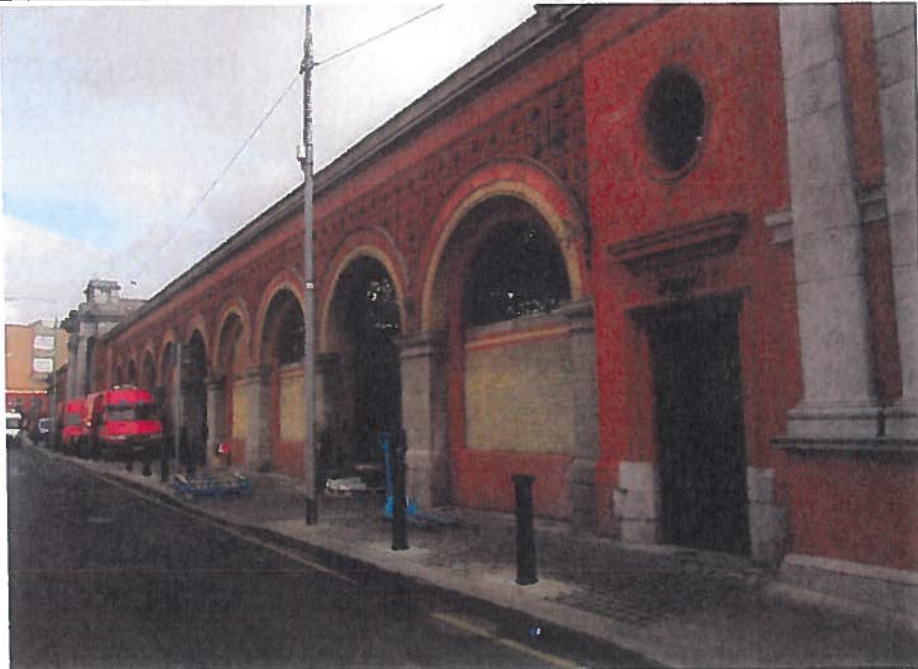
Fig 27 Arcaded façade to St Michan's Street – the general style of treatment may be classed as Romanesque
