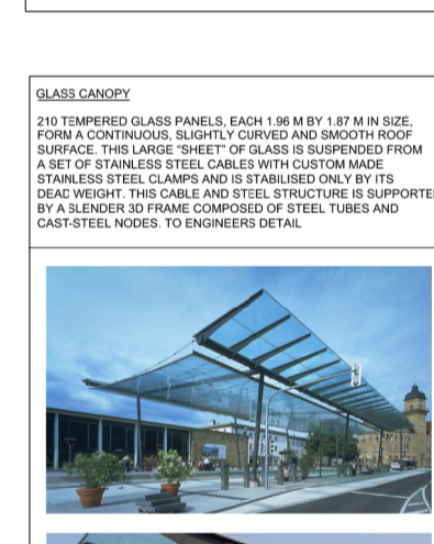
GLASS SANITY: 210 TAPERED GLASS PANELS EACH 1.8M BY 1.87 M IN SIZE. FRAME CONSTRUCTION: GALVALUM. GLASS TO BE SUPPLIED FROM A SET OF STAINLESS STEEL CLAMPS WITH CUSTOMER MADE STAINLESS STEEL CLAMPS AND IS STABILIZED ONLY BY ITS OWN WEIGHT. STAINLESS STEEL CLAMPS ARE SUPPORTED BY CAST STEEL BEAMS. CLAMPS TO BE DESIGNED TO ENGINEERS DETAIL.
