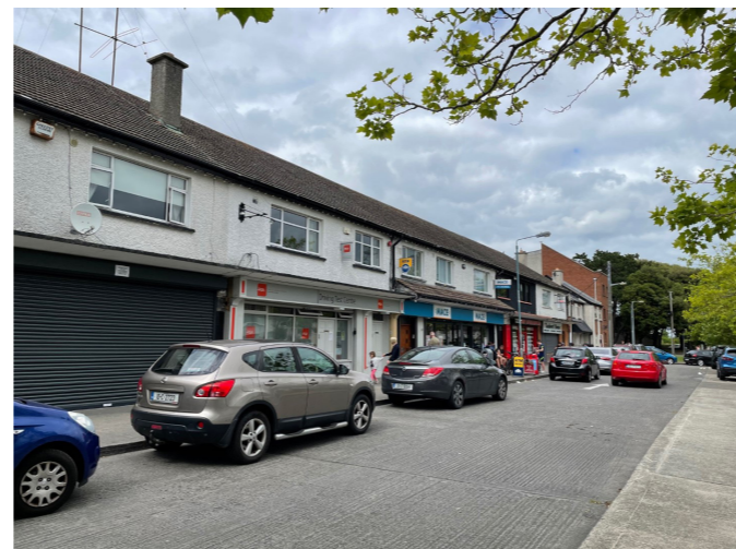
Rear condition of houses to the south of Laneway
