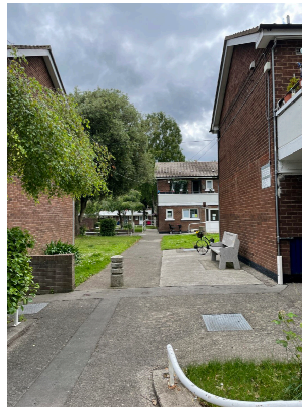
View of Pathway through the center of the site with memorial bench
