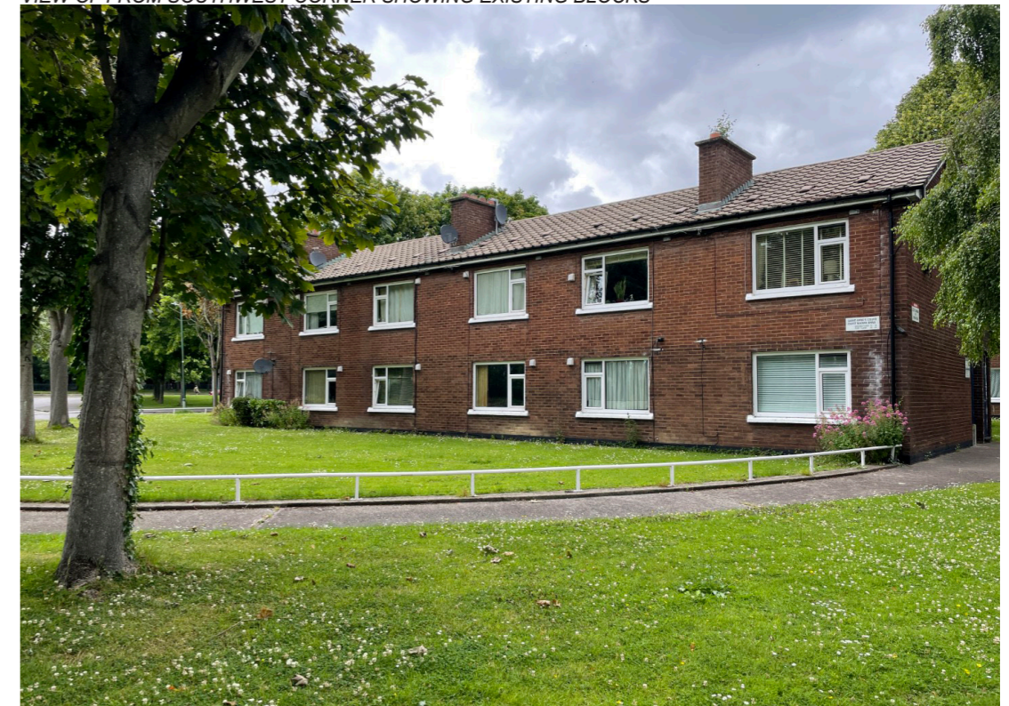
VIEW OF FROM SOUTHWEST CORNER SHOWING EXISTING BLOCKS
