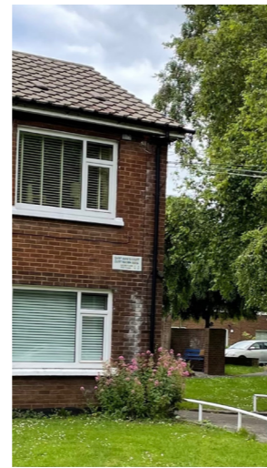
Existing facade of St. Anne's court block
