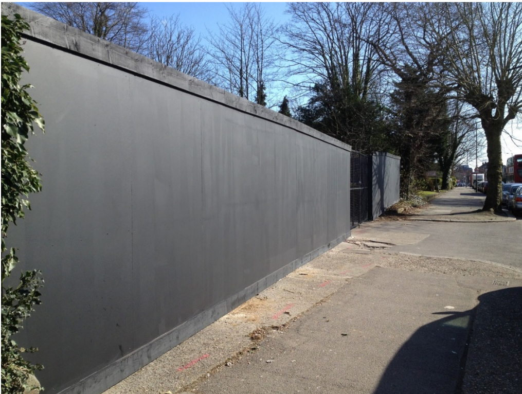
Figure 4 Sample detail of site perimeter hoarding
