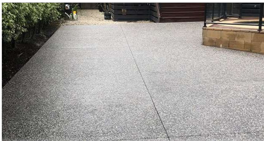
Polished concrete with exposed aggregate finish
