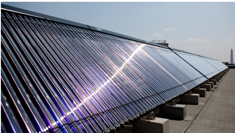
Figure 6 Solar Water Heating Panels example
