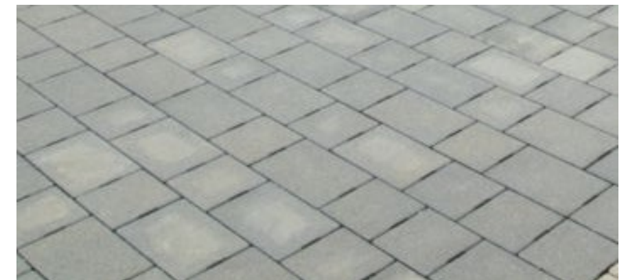
3. concrete block paver for accessible parking bays
