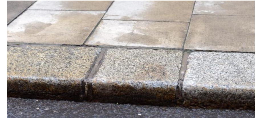
1. re used wide granite kerbs and concrete pavers
