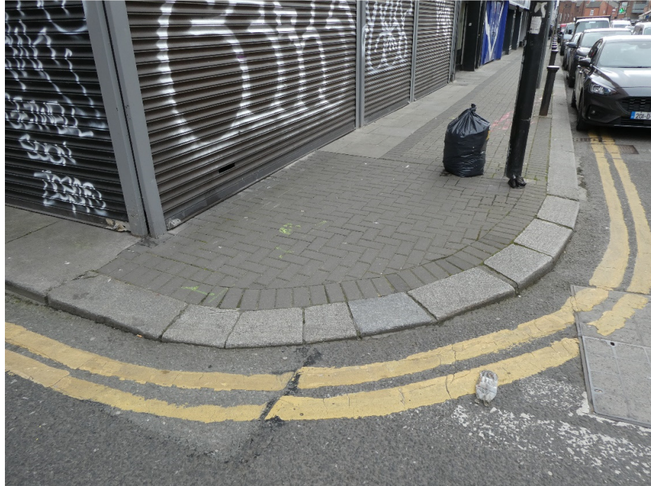
Figure 17: Junction with Engine Alley looking south along east pavement
