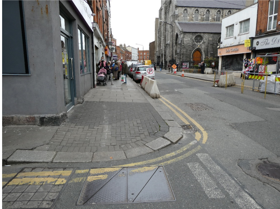
Figure 11: View from junction with Earl Street South looking north towards St. Catherine's Church
