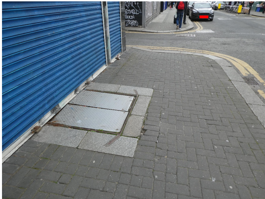
Figure 16: Junction of Engine Alley and Meath Street with stone surround to cellar opening
