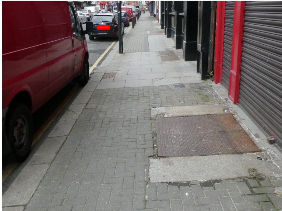
Figure 22: East pavement between Carman's Hall and Crostic Alley looking north
