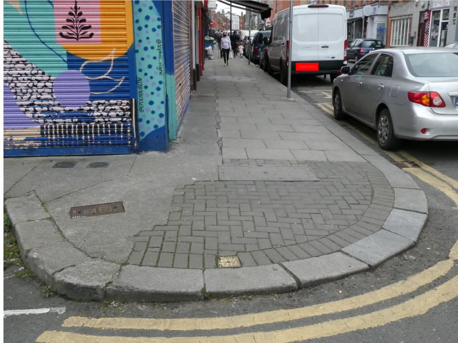
Figure 23: Junction with Gray Street looking north
