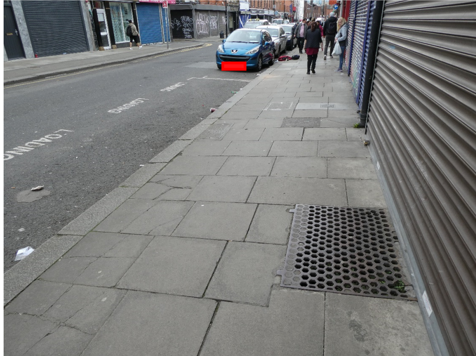
Figure 15: West pavement between Earl Street South and Meath Place looking south
