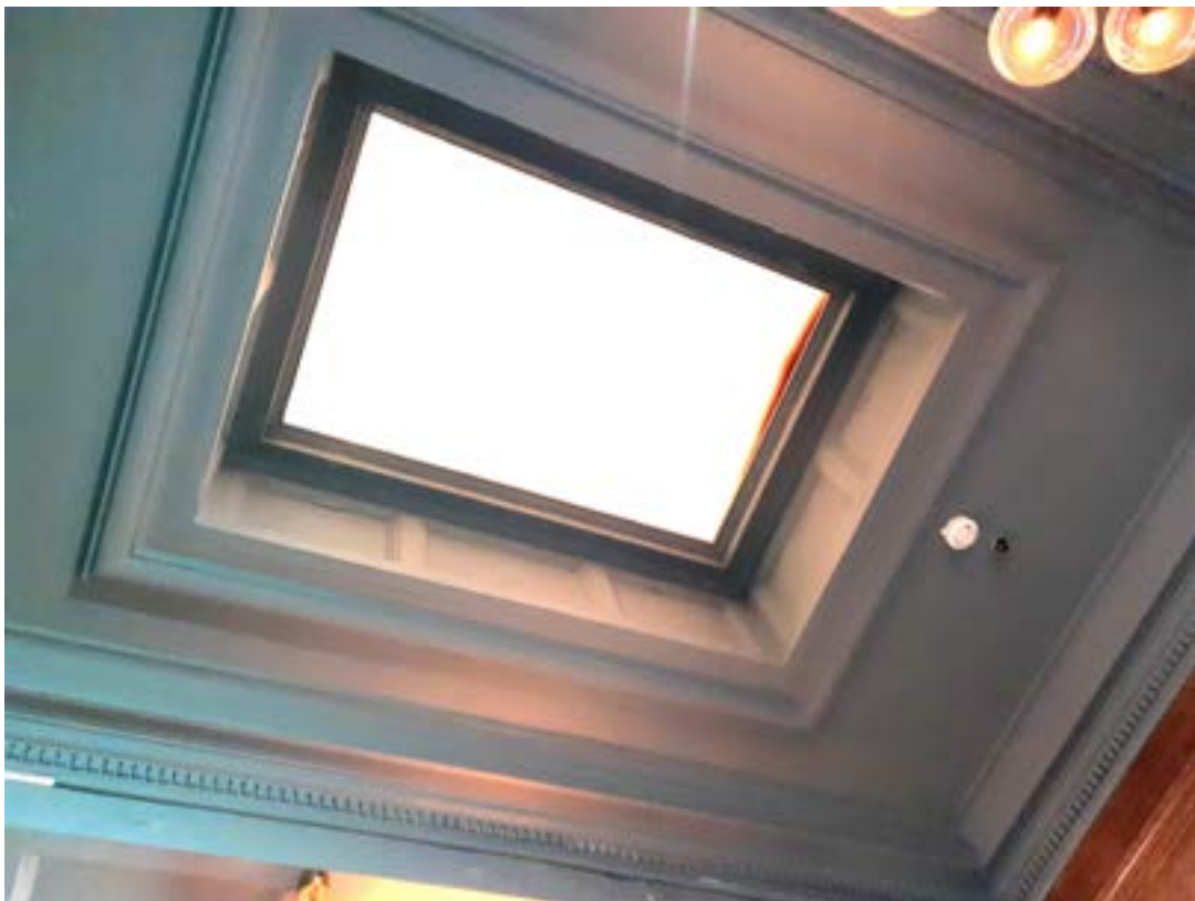
Fig. 4.25 Typical ceiling bay and rooflight in Entrance Vestibule
