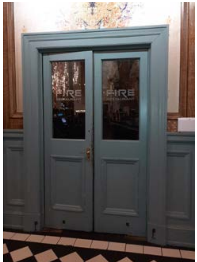
Fig. 3.42 Existing doorset to Supper Room, viewed from the existgin Entrance VEstibule
