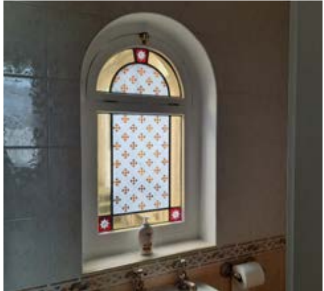
Fig. 4.46 Existing window located along southern external wall to en-suite of first floor bedroom.
