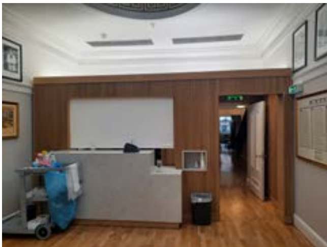
Fig. 4.42 Existing modern bar installed in the Rear Hall of the Mansion House
