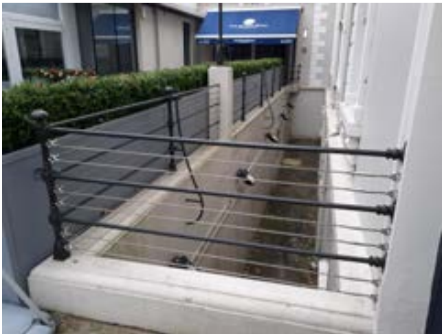
Fig. 4.8 Sections modern stainless steel wire span between the vertical uprights.
