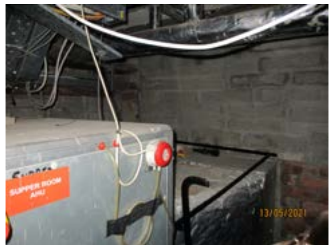
Fig. 4.60 Modern concrete walls and plant equipment beneath vestibule.
