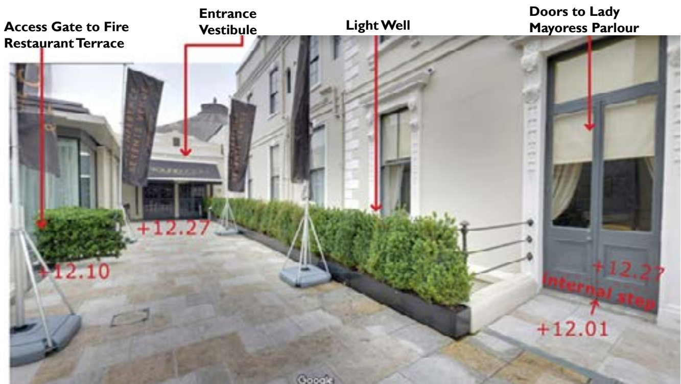
Fig. 2.3: Different levels to be accommodated in the solution – Entrances to The Parlour, The Round Room and The Oak Room as well as the exit from the adjacent Restaurant's terrace
