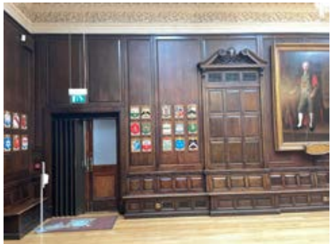
Fig. 3.37 Northern Wall of Oak Room. Doors (and fire Shutter) to existing Vestibule in LSH of image.
