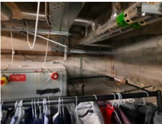
Fig. 4.57 Modern concrete walls and plant equipment beneath vestibule.
