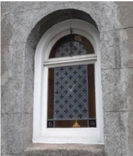
Fig. 4.40 Existing window to be removed.
