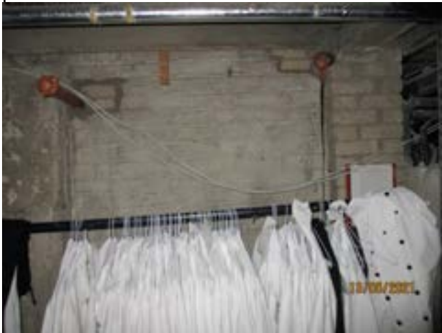
Fig. 4.55 Modern wall located in Basement Plan Room
