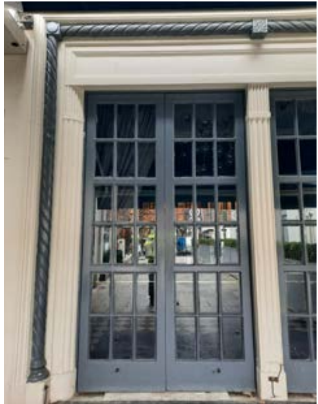
Fig. 4.3 Original timber doors inset into original opening. Decorative details surrounding doorsets.
