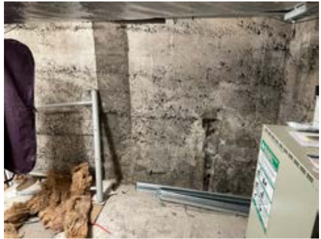
Fig. 4.56 Modern cast in-situ concrete retaining wall outside which is earth from original garden embankment
