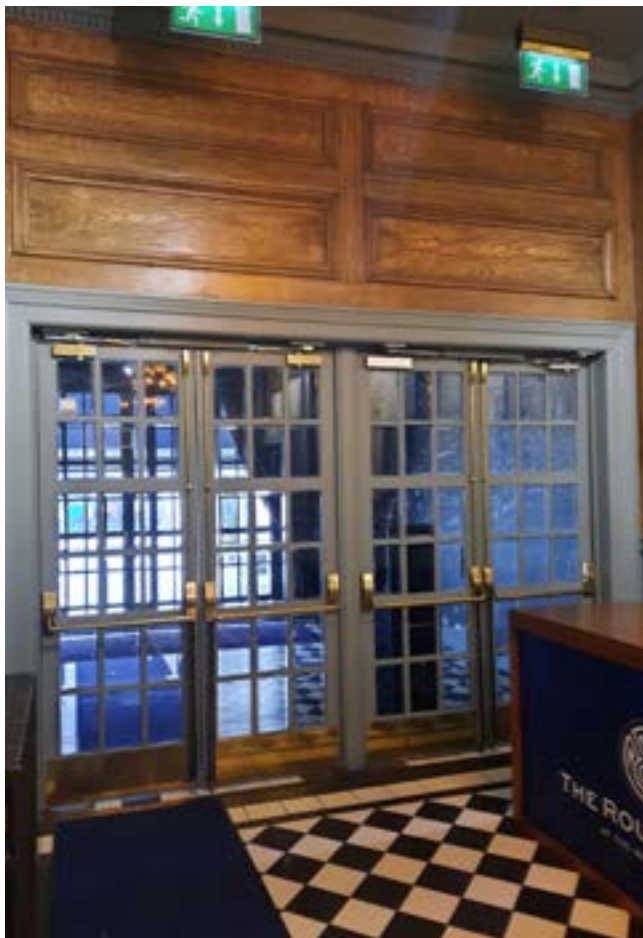
Fig. 4.17 Existing lobby door in Entrance Vestibule
