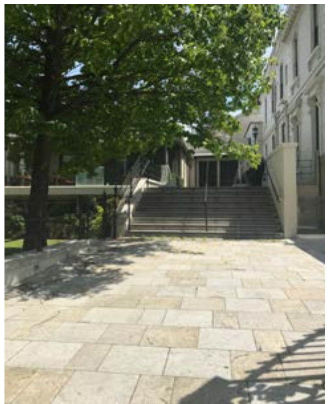
Fig. 3.22: Flight of existing steps between upper and lower areas of approach route to vestibule
