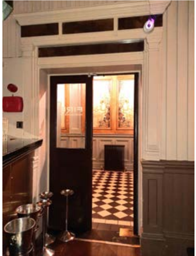
Fig. 4.32 Doorset and surrounding joinery between Entrance Vestibule and Supper Room
