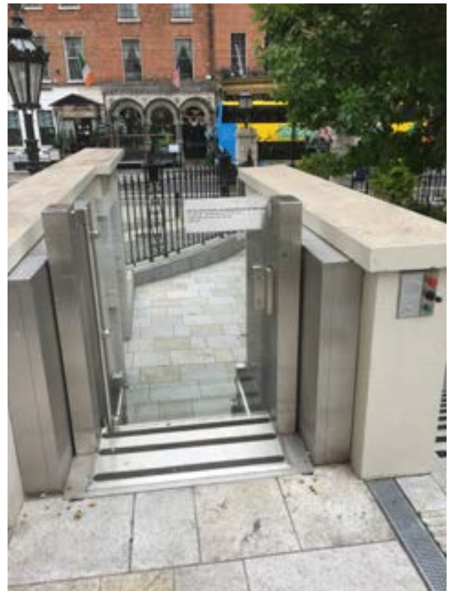
Fig. 4.16 Platform lift and flanking modern walls next to pair of doors to from Lady Mayoresses Parlour
