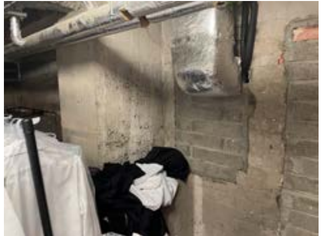
Fig. 4.59 Modern concrete wall and concrete pier at junction of Supper Room and Vestibule (basement)
