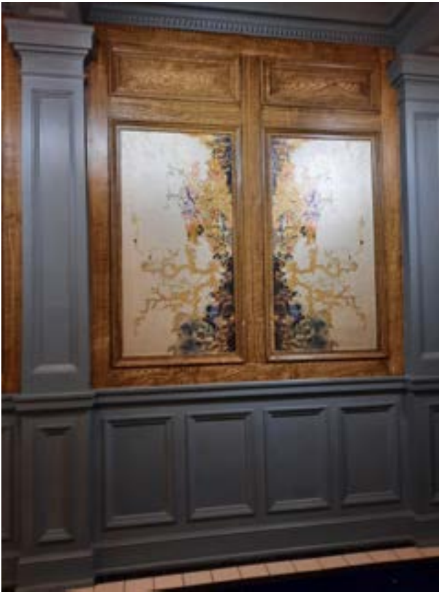
Fig. 4.20 Typical bay of Entrance Vestibule.
