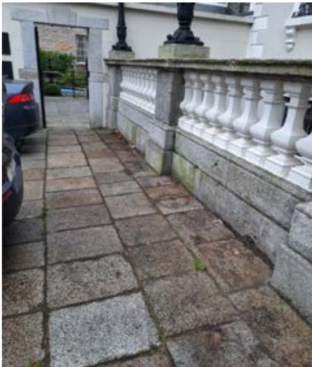
Fig. 4.14 Modern granite paving to forecourt at front of Mansion House. This paving is to be modified as part of the works.
