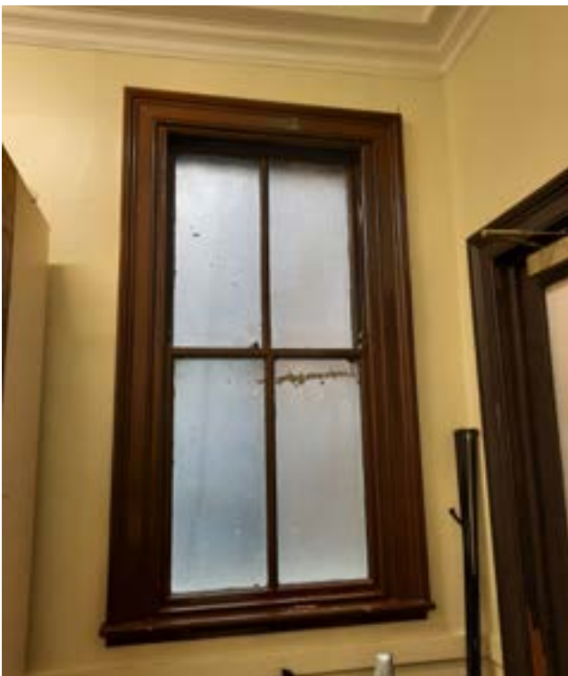
Fig. 4.27 Sliding sash window to light well from within Cloak Room
