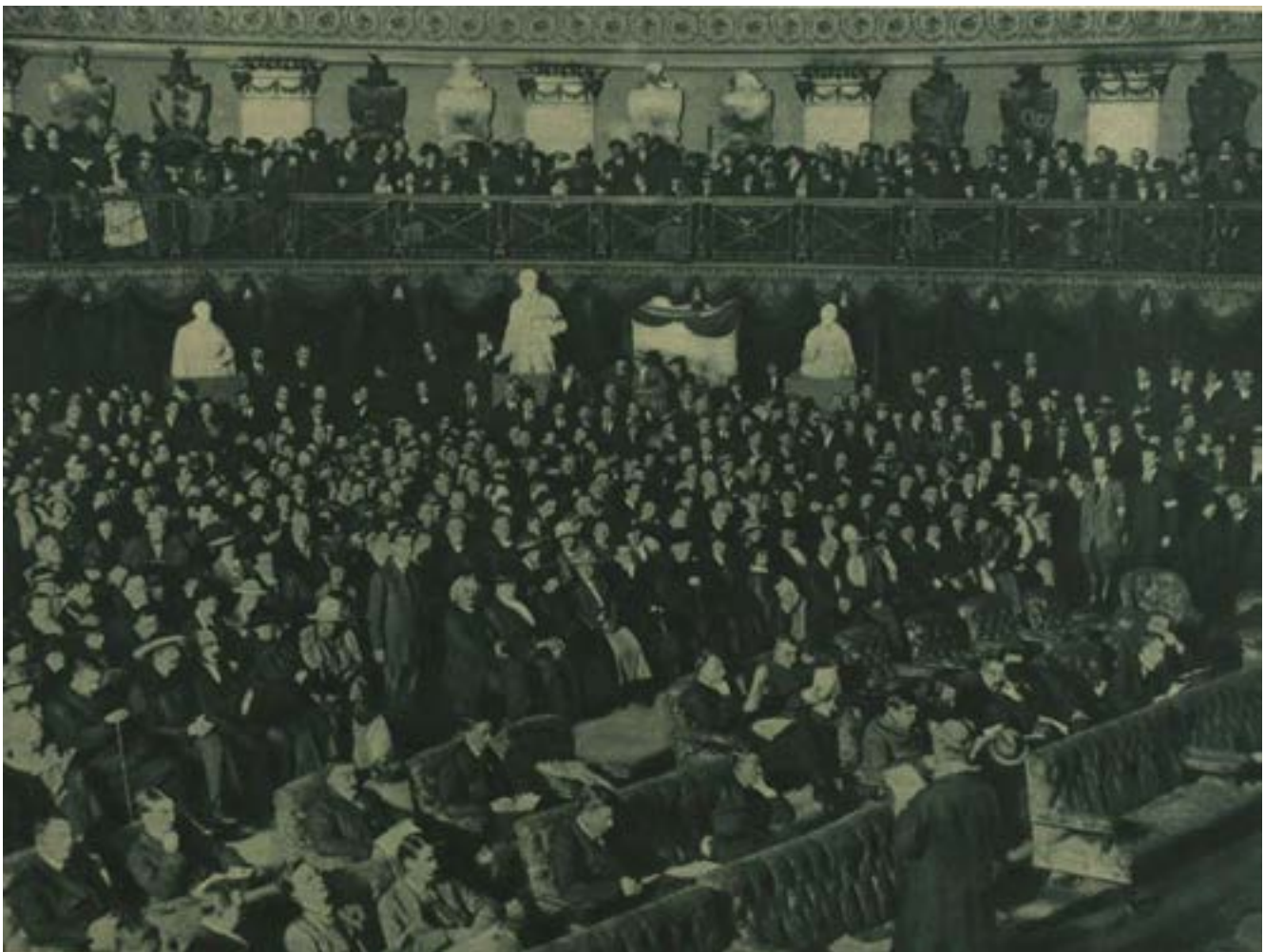
Fig. 3.40 Former interior of the Round Room
