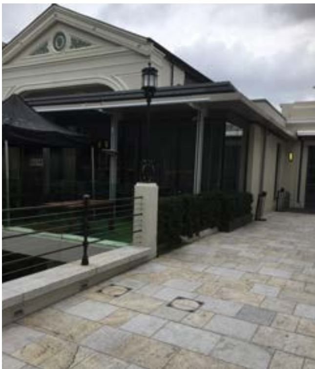
Fig. 3.24: Modern paving meets the 2012 terrace of the Supper Room
