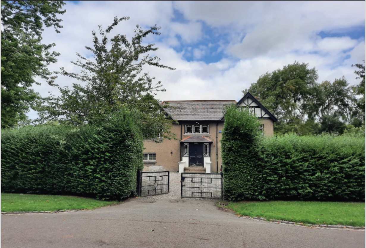
Plate 1 - CH002, facing north
