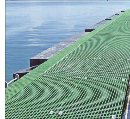
GRP ANTI-SLIP GRATING TO EXISTING BRIDGE
