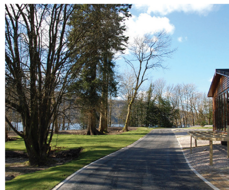
Fallbarrow Park, Windermere: Completed CellWeb TRP® Installation
