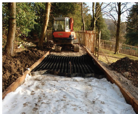
Fallbarrow Park, Windermere: CellWeb TRP® Installation
