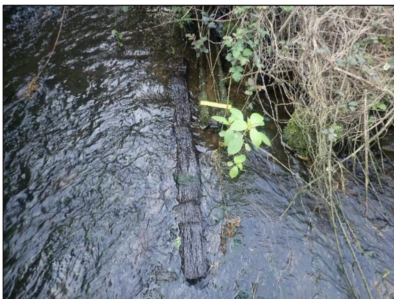
Plate 21: Oak timber and steel I-beam resting on concrete covered stone apron.
