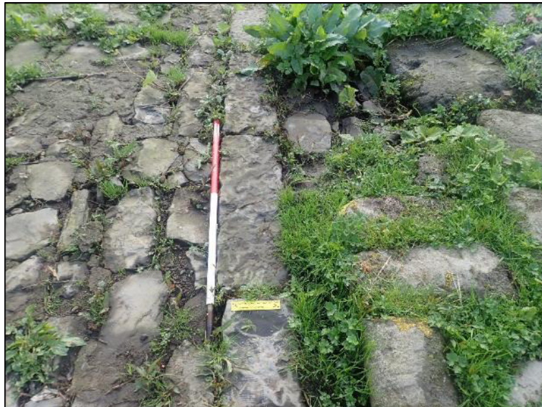
Plate 14: Weir (left) and weir sill (centre) with hessian sacks (right) (1m/ 150mm scales).
