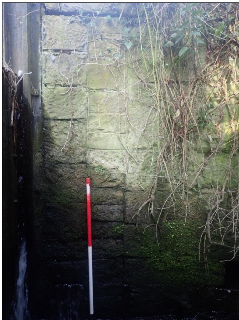
Plate 20: Masonry feature indicating the previous presence of an anchor point for the timber post of an earlier sluice gate (1m scale).
