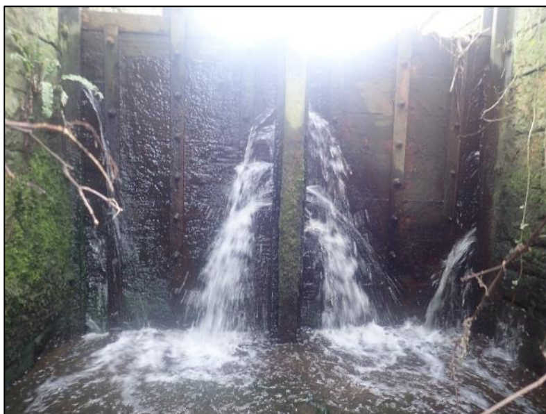
Plate 18: Downstream side of flow control sluice gate.
