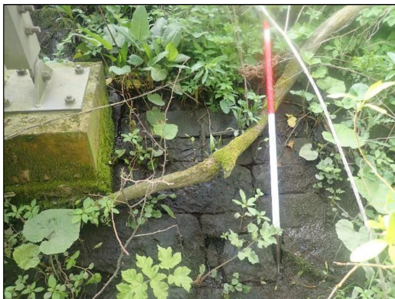
Plate 33: Concrete support of footbridge built onto weir stonework (1m scale).
