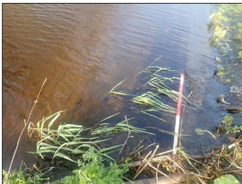
Plate 15: Ramp of weir (underwater) (1m scale).
