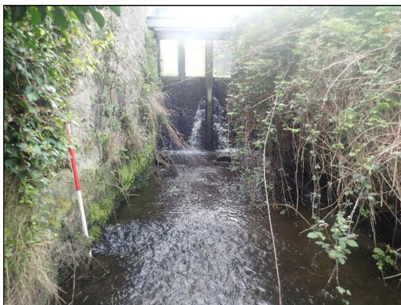
Plate 19: Sluice gate passage (1m scale).
