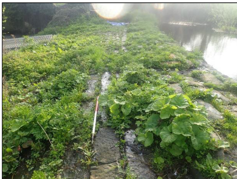
Plate 16: Dry section of weir in use as crossing point (1m scale).
