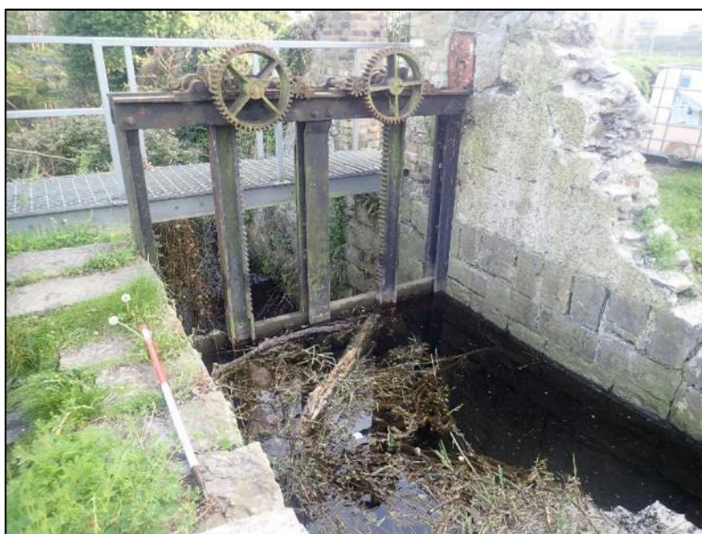
Plate 17: Upstream side of flow control sluice gate (1m scale).
