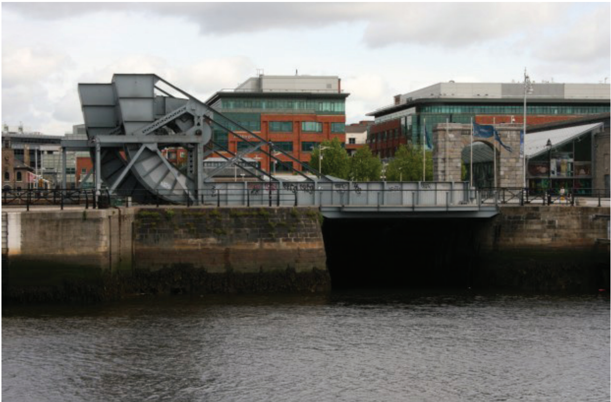
Figure 16 - Scherzer Drawbridge with arch to right
