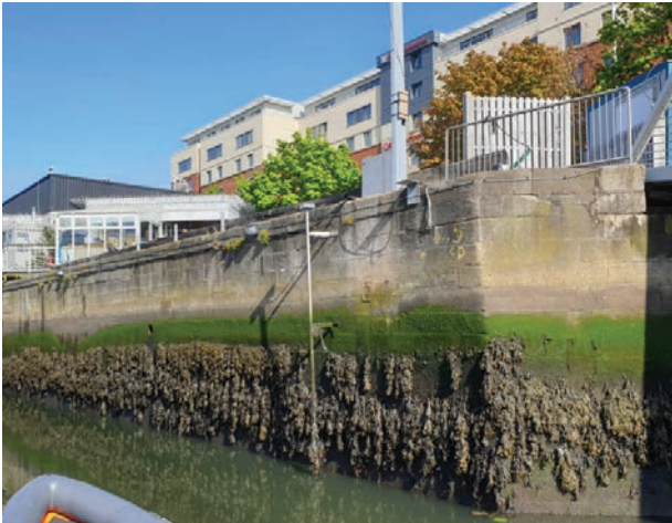
Figure 20 - Existing structure bordering Custom House Quay
