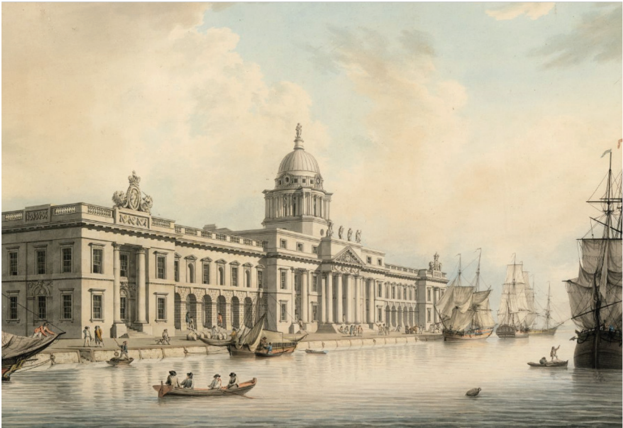
Figure 5 - James Malton's 1792 View of the Custom House
