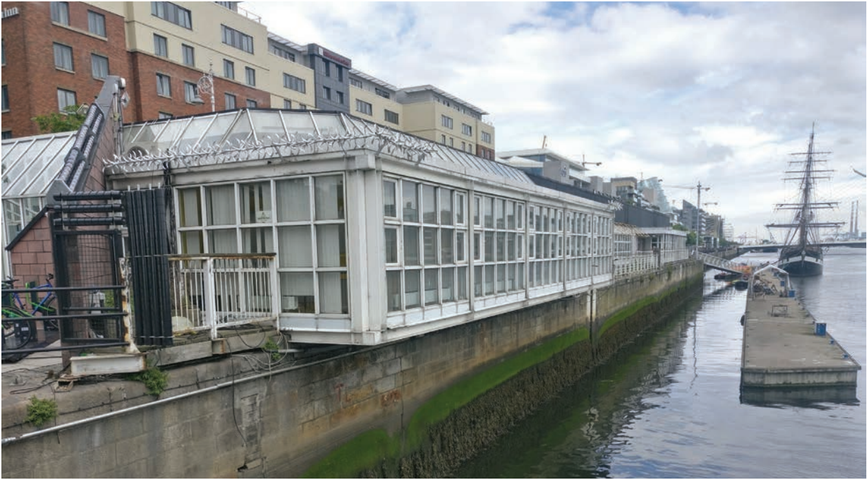
Figure 22 - Existing quay wall, building and pontoon, Custom House Quay
