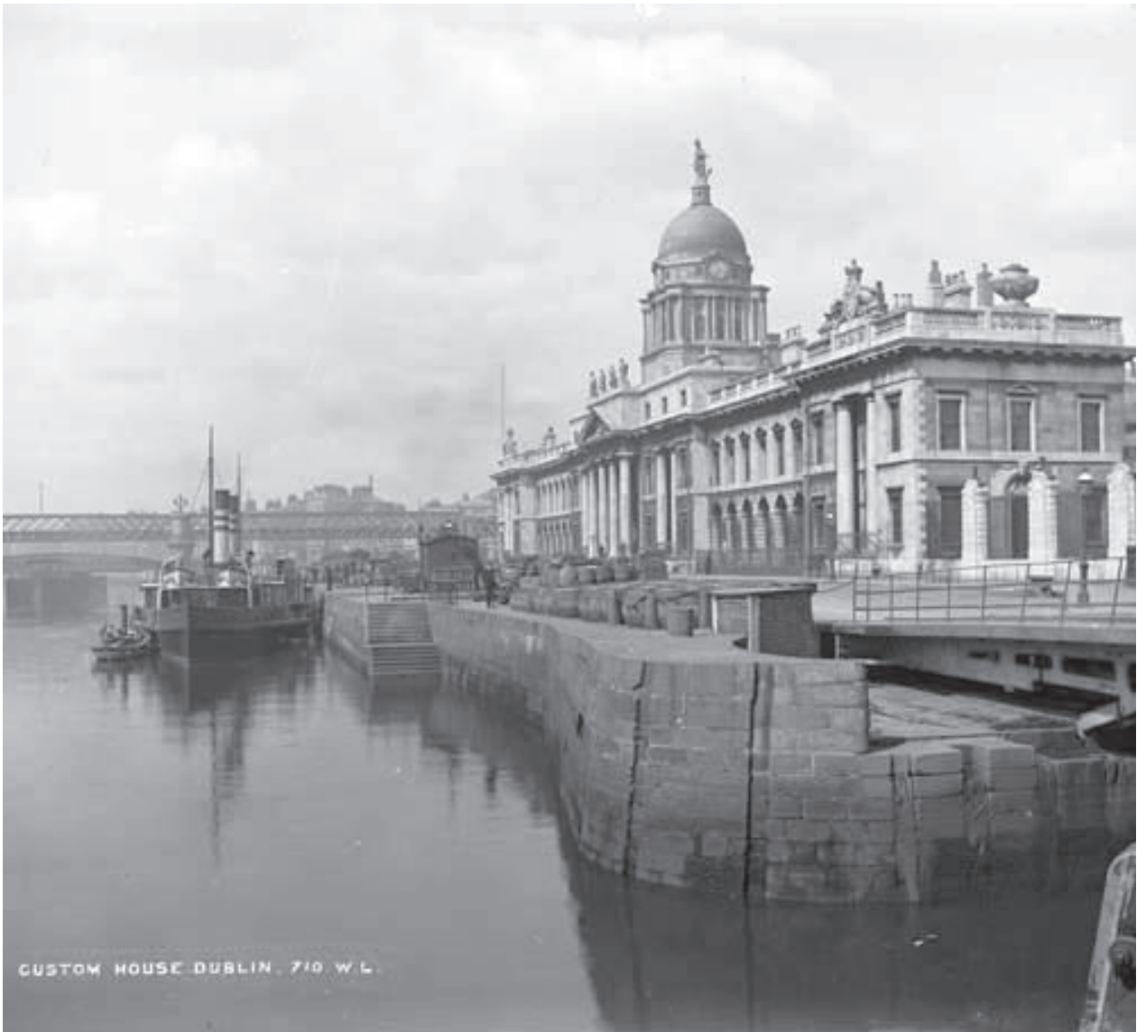
Figure 10 - View of entrance to docks (NLI Lawrence Collection c.1880-1900)
