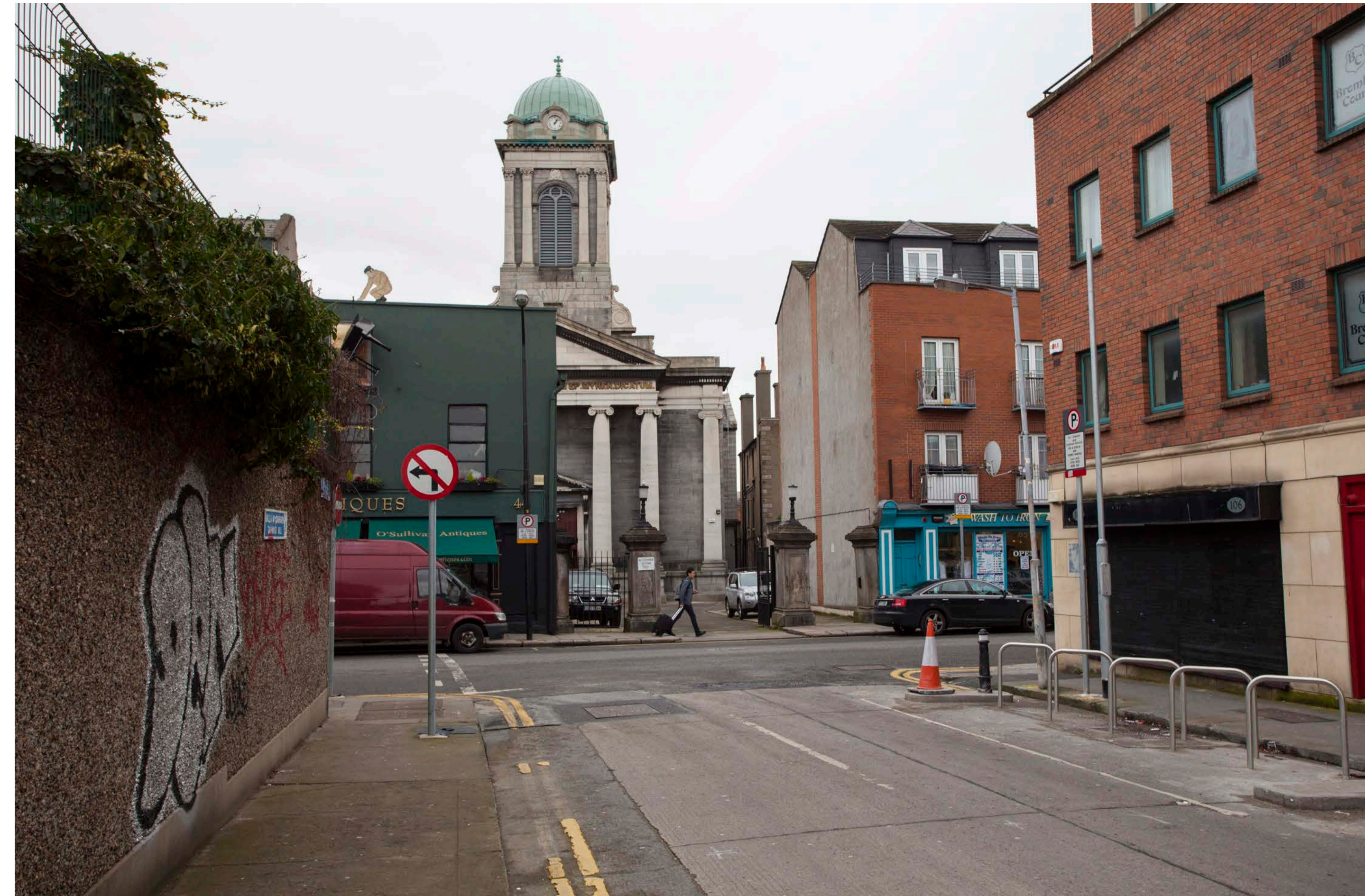
Existing view at junction of Carmanhall Road & Francis Street
