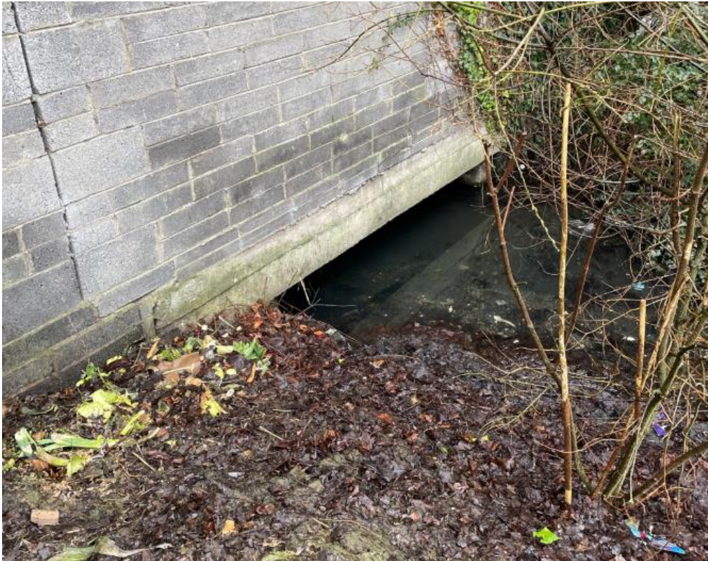
Figure 2-3 Finglas Stream Open Channel Section Outlet (Facing East)
