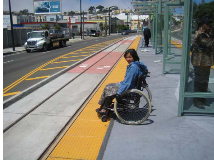
Tactile warnings protect blind persons – and all other passengers – from getting too close to the platform edge in transit stations.
