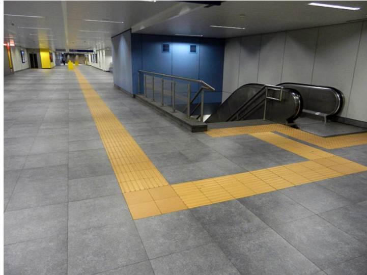
Routing for vision-impaired people by ridges/grooves in the pavement.
