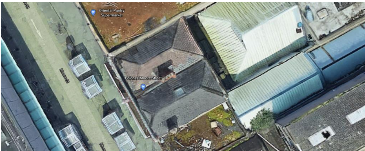
Fig. 7: 20/21 Moore Street showing early roof form perpendicular to street with hipped sections to front and rear (Google Earth 04/12/20)
