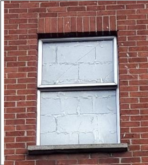
Fig. 5: First floor window opening with modern frame
