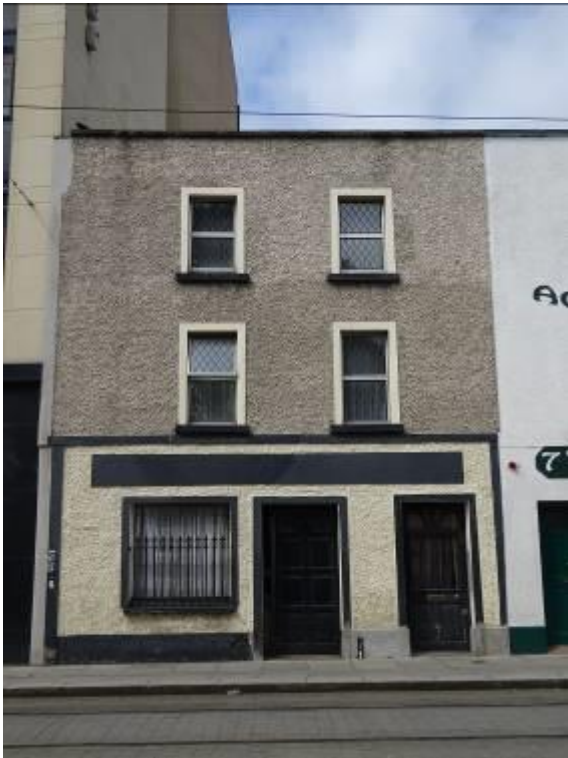
Fig.3: Principal/south elevation. Note the disproportionate ratio of solid to void to the elevation indicating an early construction date.
