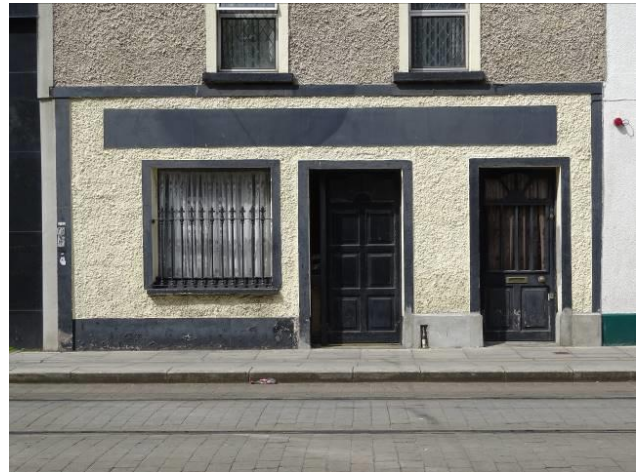
Fig.7: Detail of former shopfront to ground floor. Note the separate access to residential accommodation and rendered fascia board.
