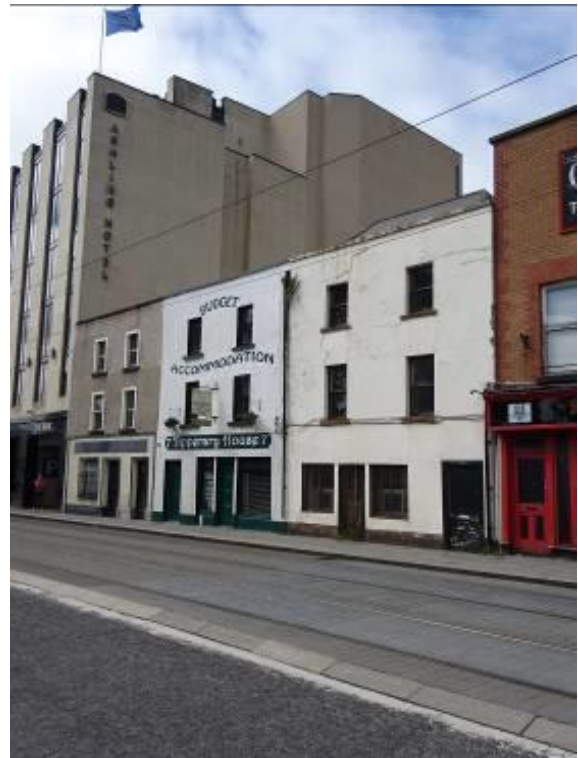
Fig.4: Context view of No.6 (right), No.7 (centre) and No.8 (left) Parkgate Street taken from the east showing the properties now dominated by the Ashling Hotel.
