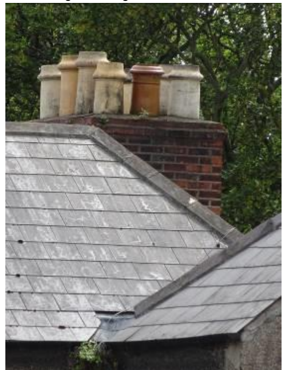
Fig.7: Detail of substantial chimney stack shared with No.6 Parkgate Street.
