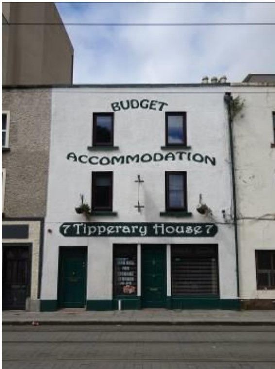
Fig.3: Principal/south elevation. Note the disproportionate ratio of solid to void to the elevation indicating an early construction date.
