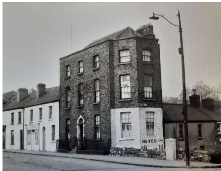
Fig. 5: Archive photograph of No. 31 Old Kilmainham (source Irish Architectural Archive, ref. 2001/051-PH 202).
