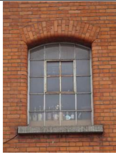
Fig. 10: Metal window, north elevation
