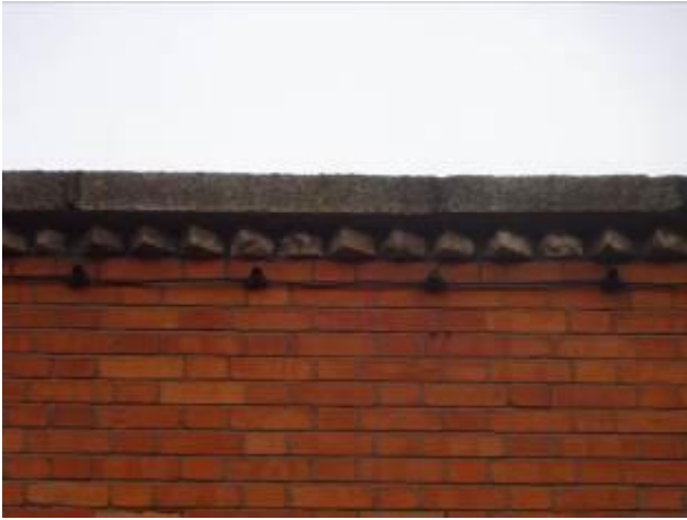
Fig. 9: Dogtooth course, north elevation
