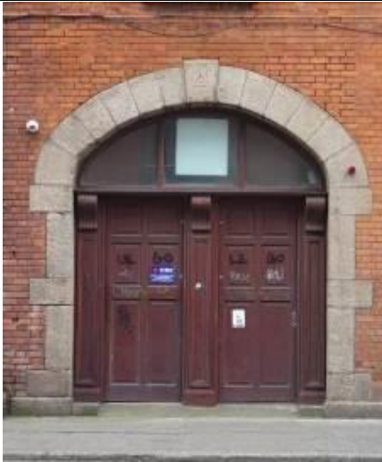
Fig. 11: Former goods entrance, north elevation
