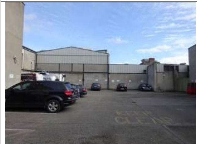
Fig. 7: West elevation of N-S running section of building along Bow Street
