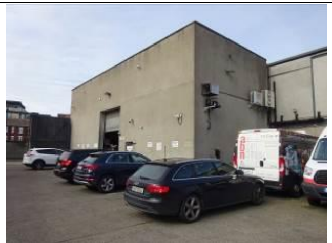
Fig. 8: View of west end of building from southeast
