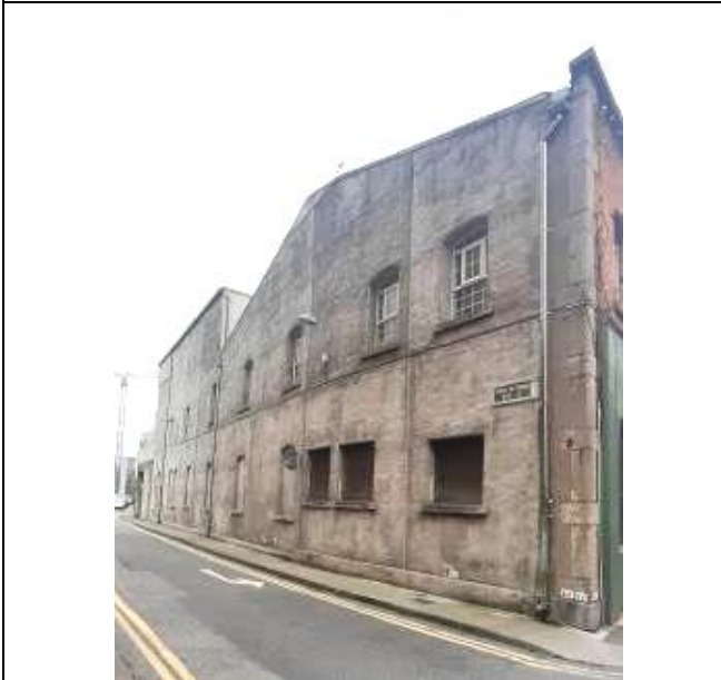
Fig. 5: East elevation from northeast
