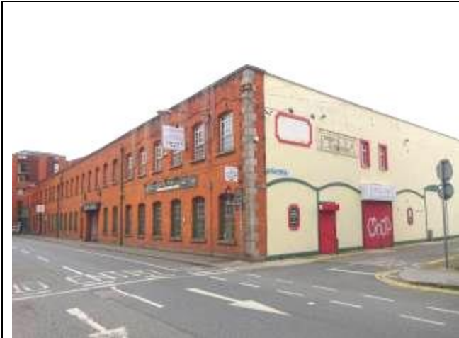
Fig. 3: View from northwest
