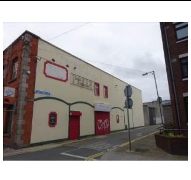
Fig. 6: West elevation from northwest
