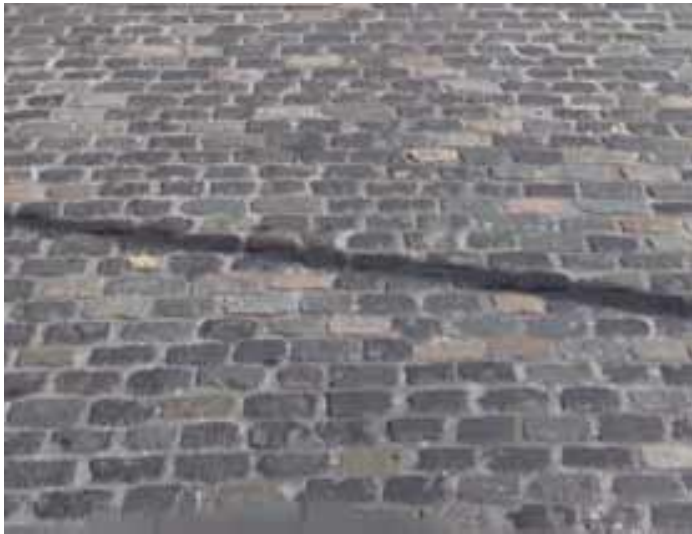
Fig. 15 Re-laid Dublin cobbles in May Lane
