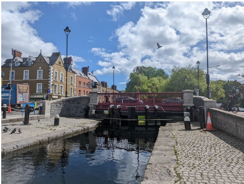
Plate 12: La Touche Bridge (DCIHR Structure), facing northeast
