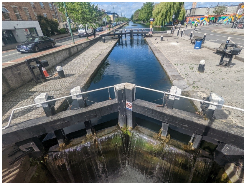
Plate 14: Canal Lock (DCIHR Structure) facing west
