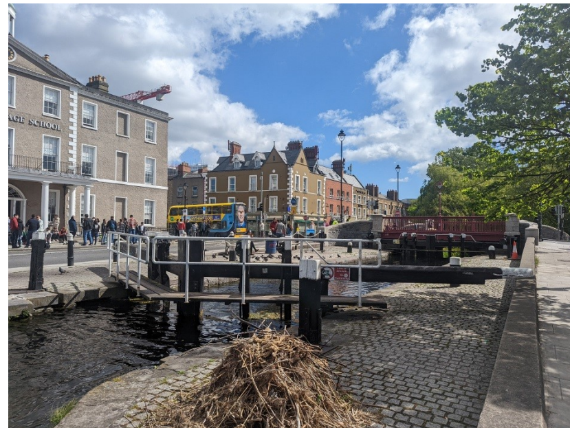
Plate 13: Canal Lock (DCIHR Structure) facing northeast.
