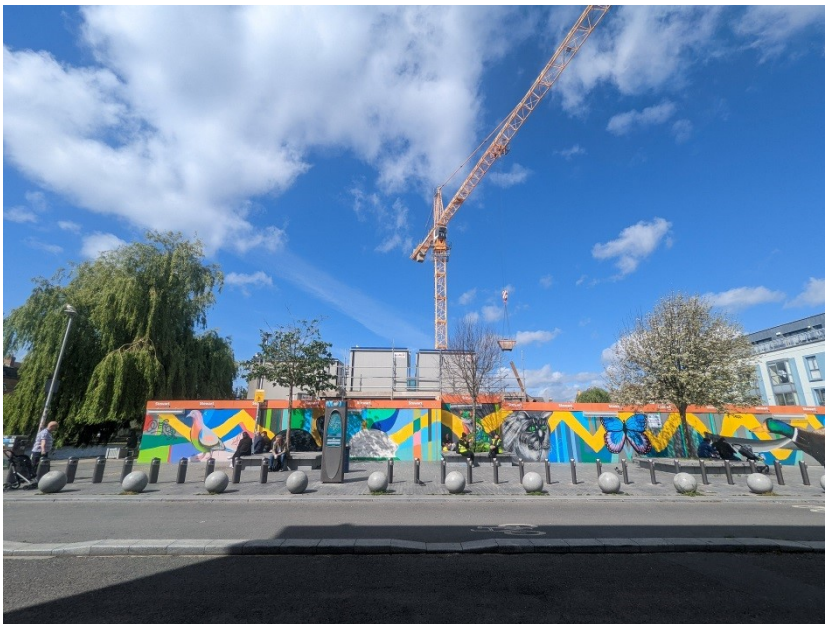
Plate 7: Site overview, facing west.
