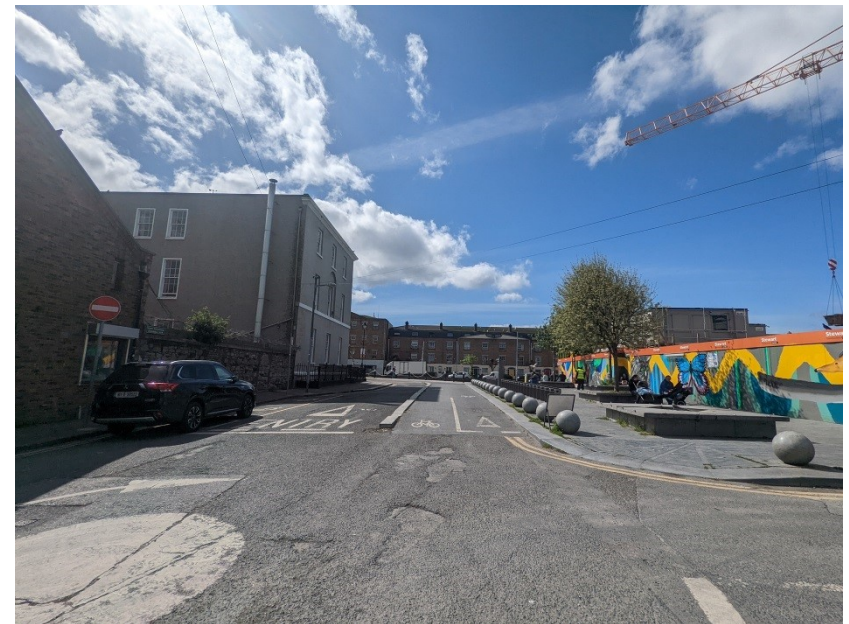
Plate 8: View along Richmond Row, site to the right, facing south.
