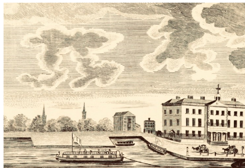
THE GRAND CANAL HOTEL & PORTOBELLO HARBOUR
