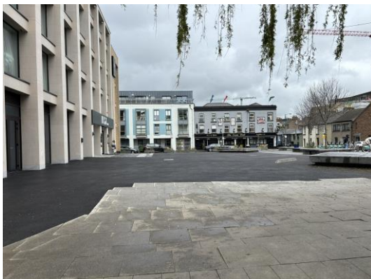
View north towards the Lower Deck Bar
