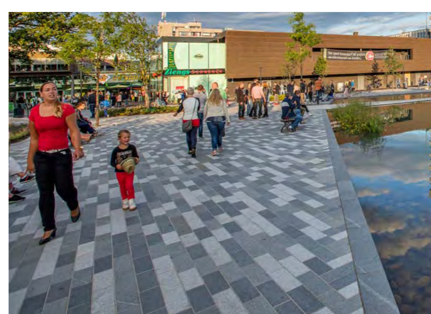
Stone paving; new and reused
