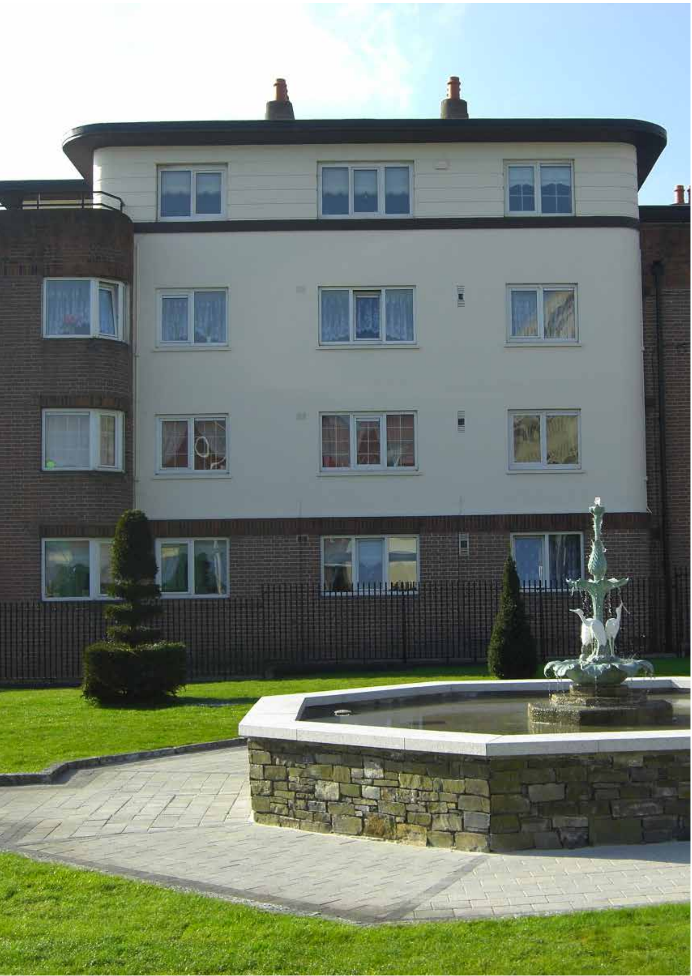
Chancery Street House and Chancery Park
