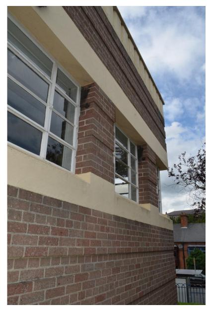
Fig. 12B – East Façade, close up of steel window recesses. Circa 50mm diameter drilled holes in window reveal brick.
