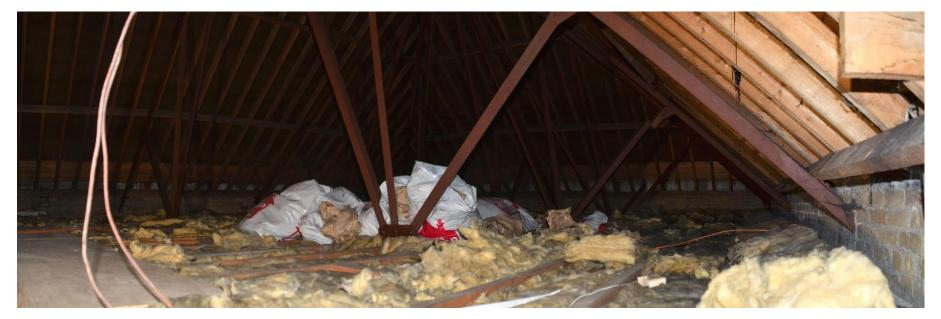
Fig. 26A - Above — Attic view east from trapdoor. Traditional rafter roof with dated sarking felt on timber purlins and steel truss structural framing.
