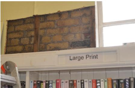
Fig. 19A – Above – Corner steel window from inside with cantilever structural ringbeam over.
