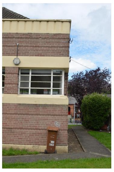
Fig.10A - Rear corner detail east with corner steel window, patterned recessed brick bands, concrete base, cill, lintol and parapet courses. Vents to raised floor.
