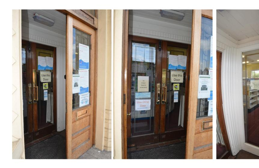
Fig. 14A, B & C – Entrance Lobby Arrangement – Narrow space, glazed sides, polished brass ironmongery, low ceiling with emergency lighting added, fluted art deco detailing on inner wall. Glazed natural timber doors.
