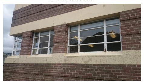
Photo 9: Elevation detail, note damaged window frames
