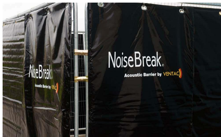
Figure 16: Temporary Construction Noise Barrier © Ventac
