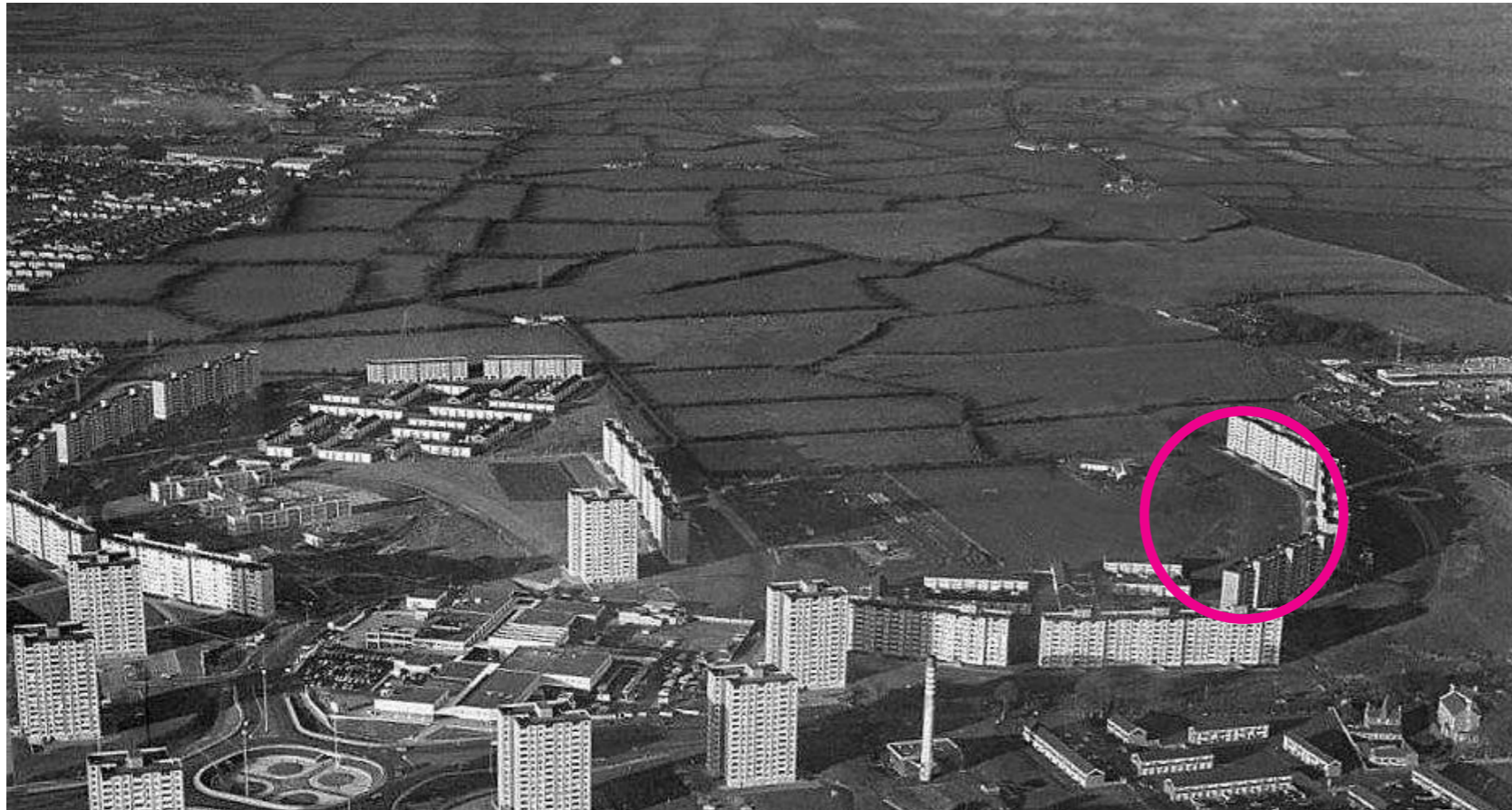
Image 12 - Aerial View of Site in 1970
