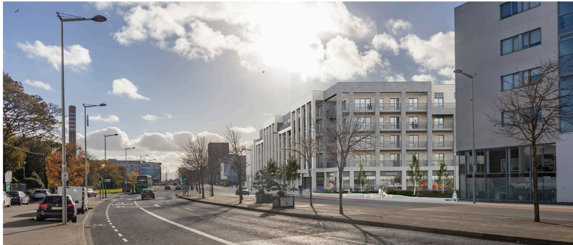
Image 39 - Site 5, Viewed from the north along Ballymun Road, at its corner to St. Pappin's Square
