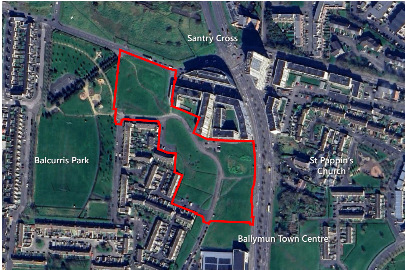
Image 5 - Site Aerial Photo
