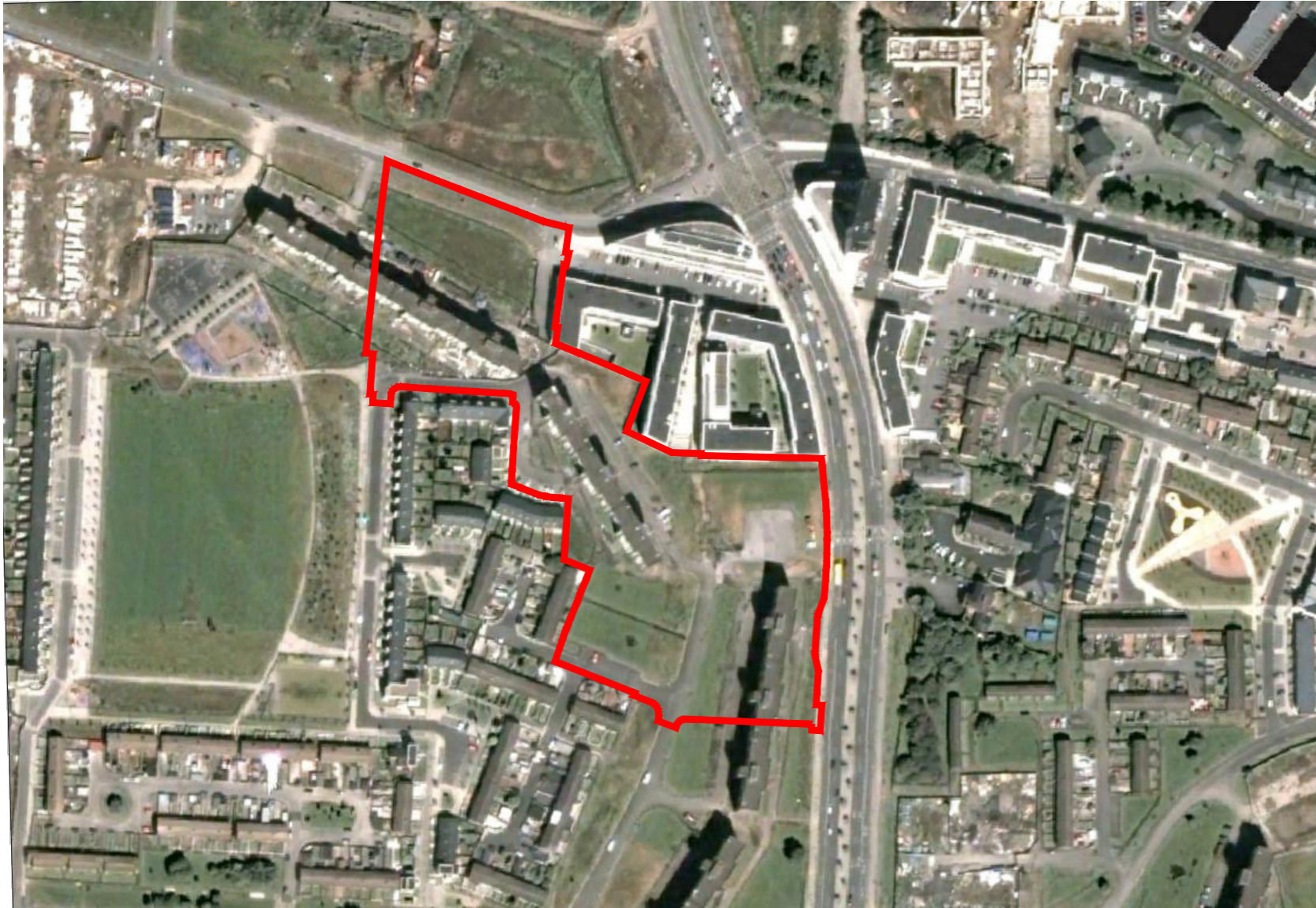
Image 16 - Aerial View of Site in 2008
