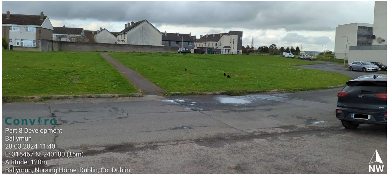
Figure 8.1: Outline Proposed Waste Compound, Quarantine Area, Temporary Soil Stockpile Storage, Material Storage Area, Dedicated Refuelling Area in the central area of the site.
